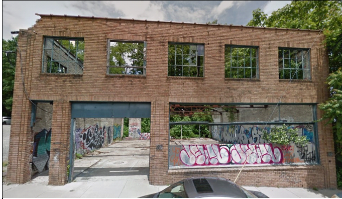
EXISTING BUILDING STRUCTURE
