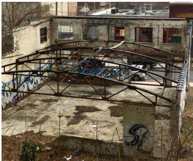
EXISTING BOWSTRING TRUSSES
