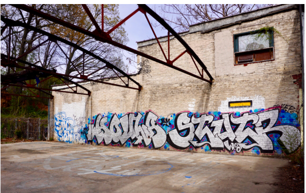
INTERIOR SPACE PRIOR TO RETROFIT
