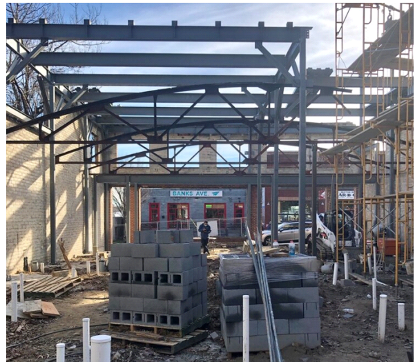
CONSTRUCTION OF ROOF DECK SUPERSTRUCTURE
