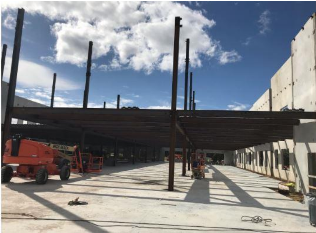
COMPOSITE STEEL SECOND FLOOR FRAMING
