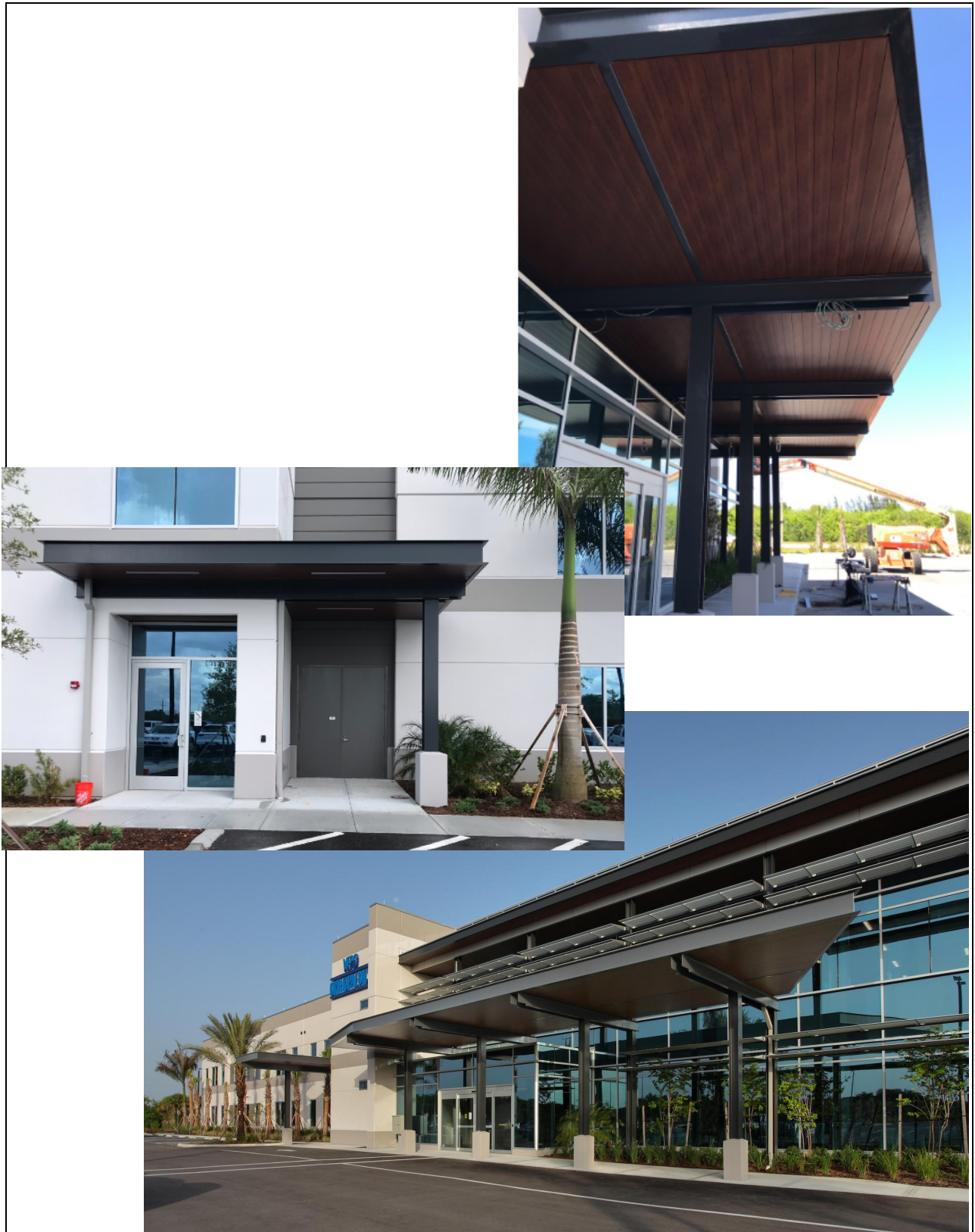
EXPOSED STRUCTURAL STEEL CANOPIES AND SUN SHADE SUPPORTS
