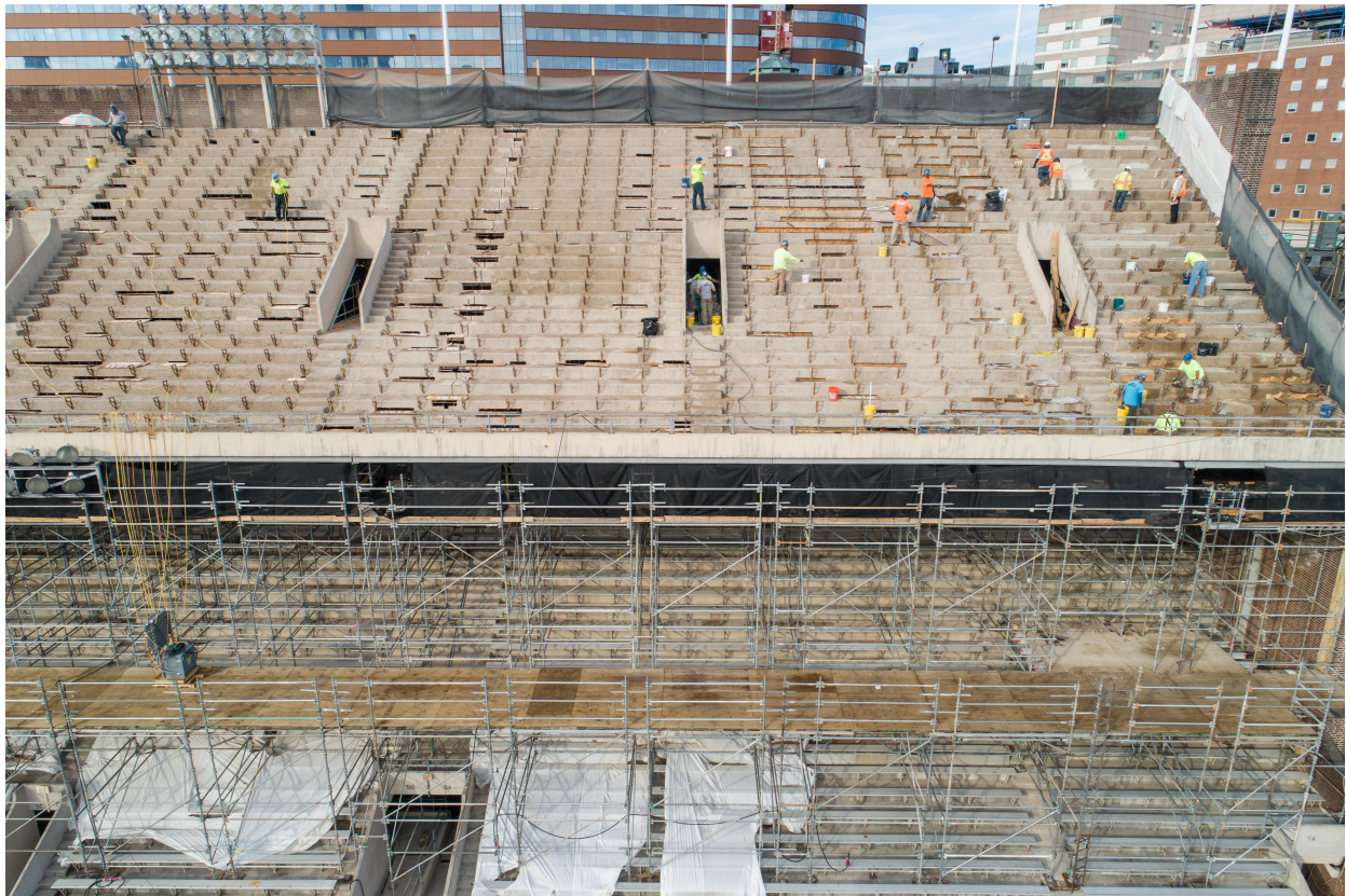
Figure 8. Repairs in process upper south grandstands.
