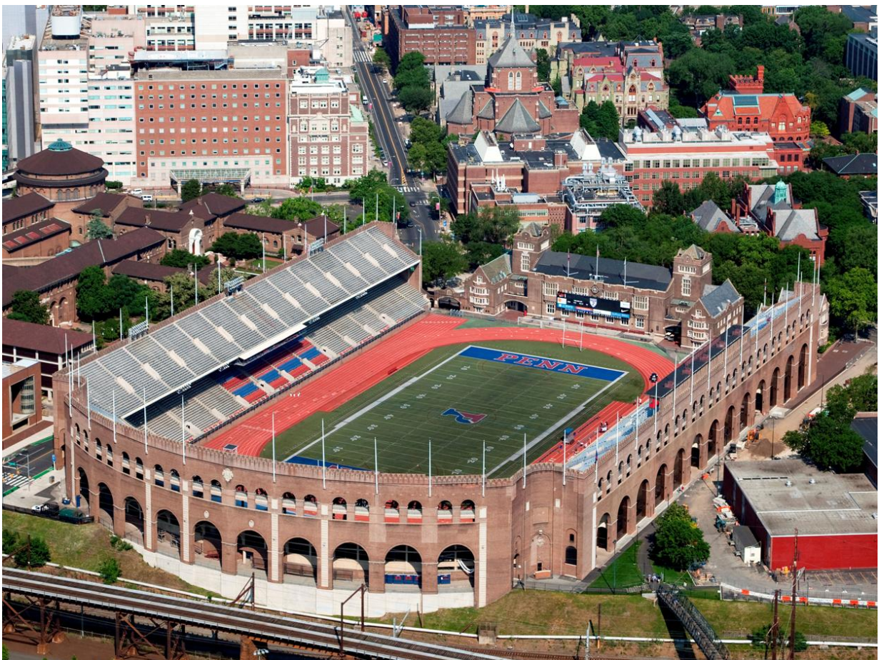
Figure 2. Franklin Field - exterior view.
