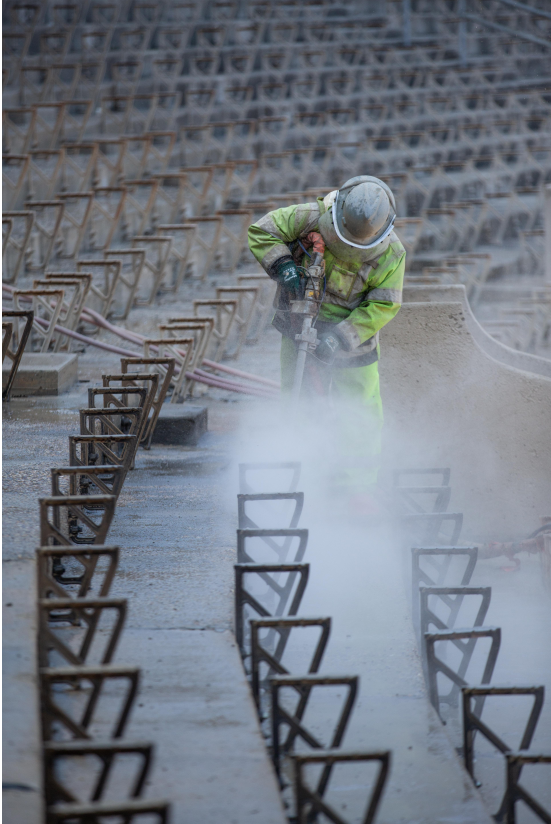
Figure 6. Existing coating removal via hydrodemolition.
