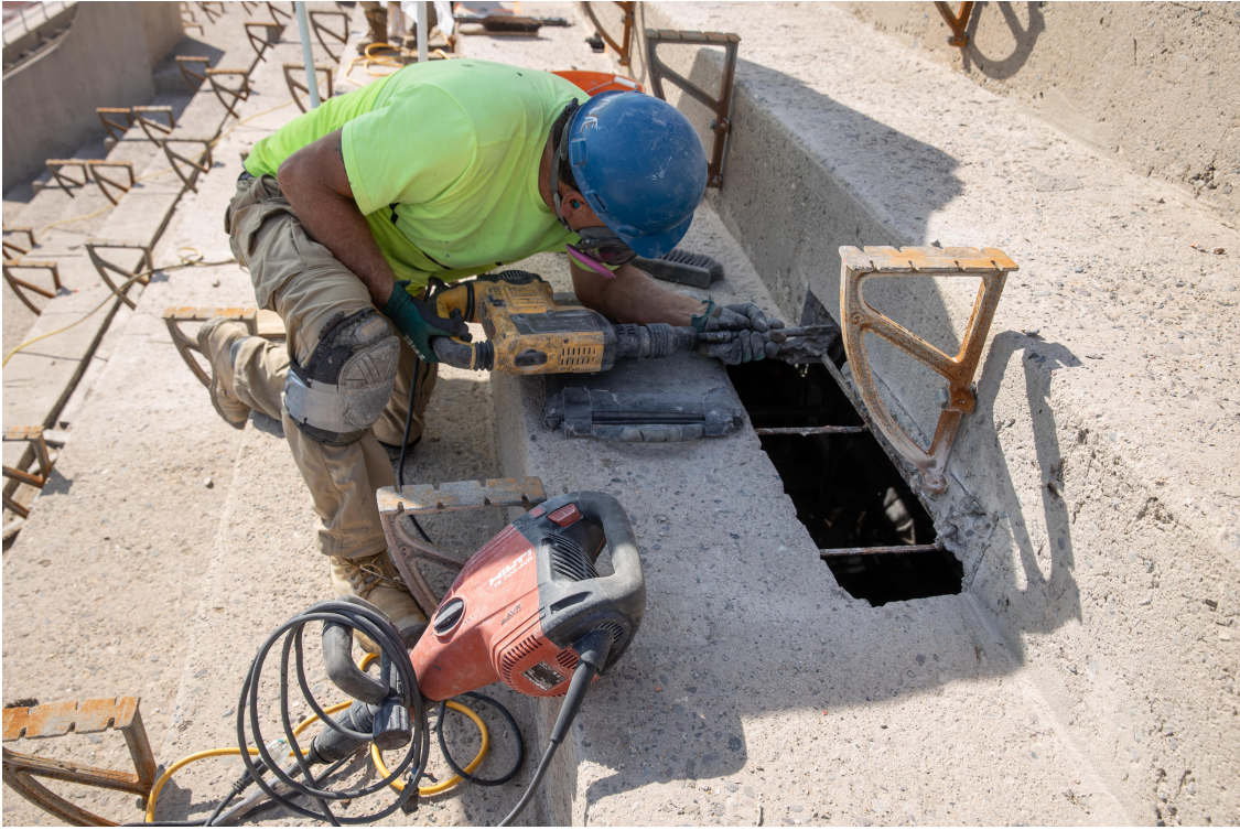
Figure 5. Full depth repair being completed.
