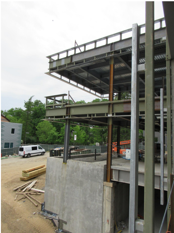
Figure 4 - Cantilevered roof at new outdoor patio space
