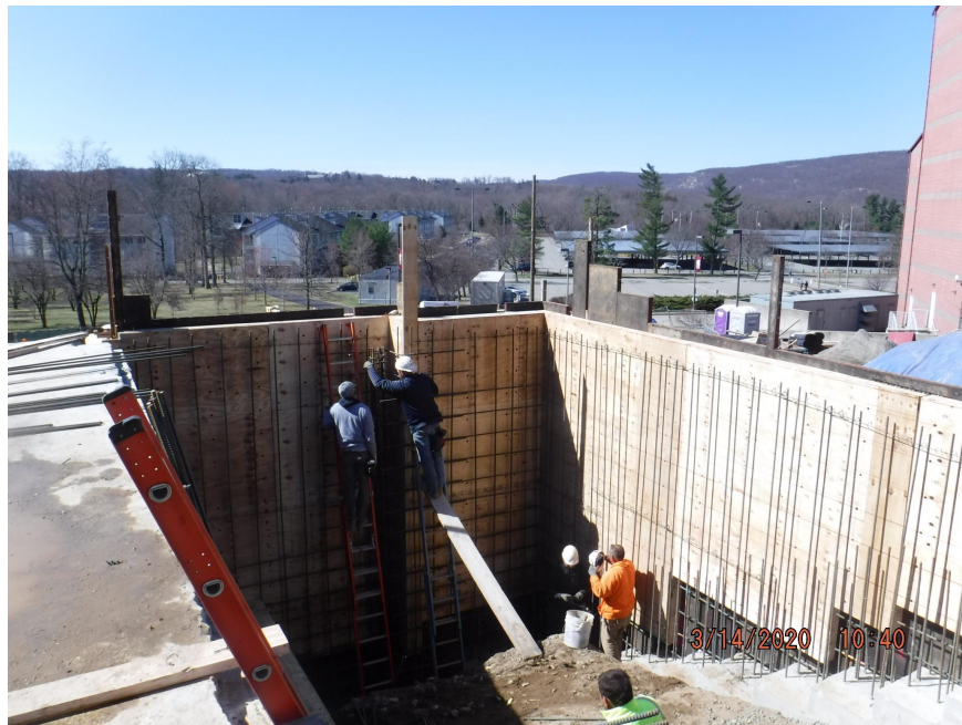
Figure 10 - Deep foundations at west balcony addition
