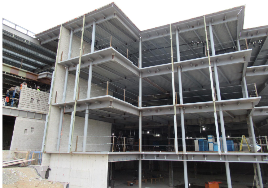
Figure 3 - New floor area at curtain wall elevation
