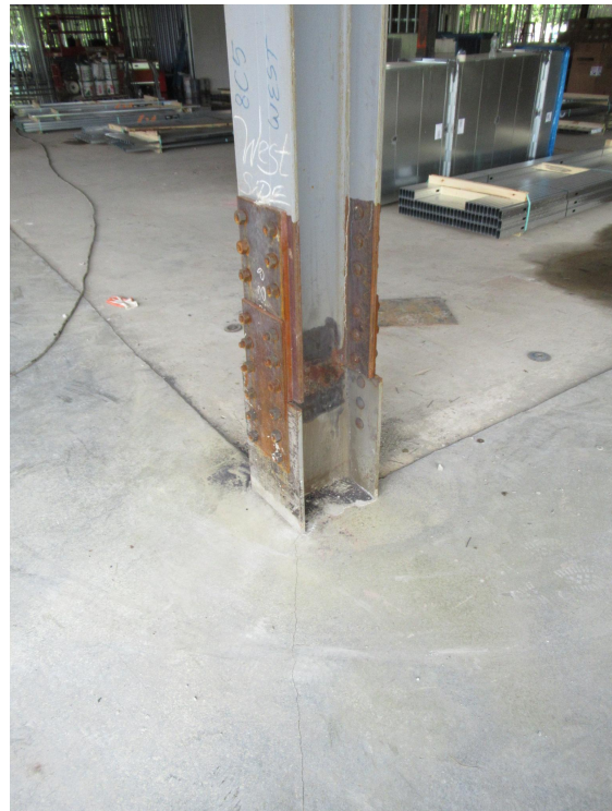
Figure 5 - Exposed bolted splice of new column piece on to existing
