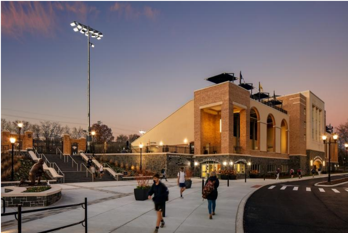
Grandstand Building Southwest Elevation with Main Entrance Grand Stair
