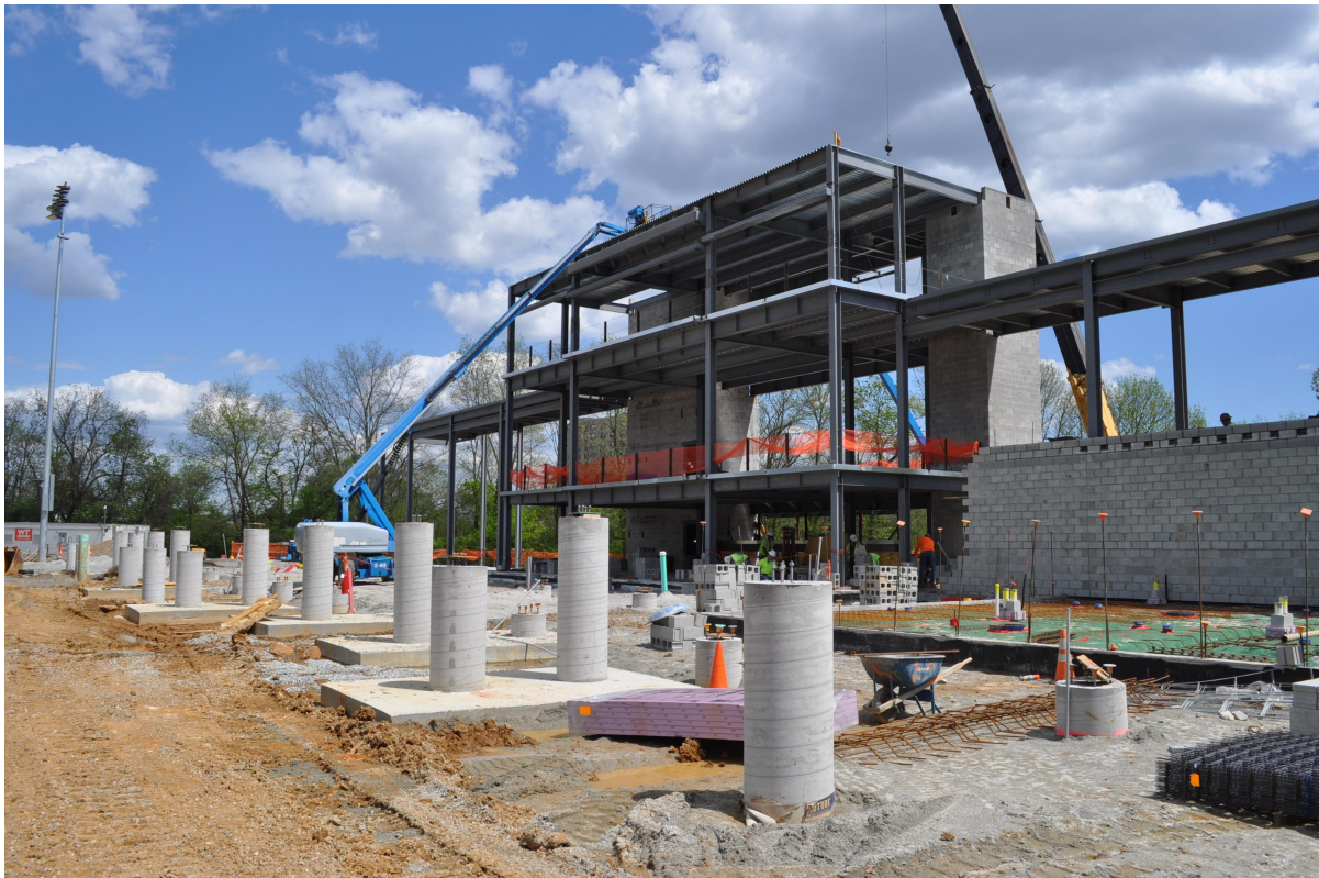
Grandstand Building Northwest Elevation Construction with Bleacher Piers
