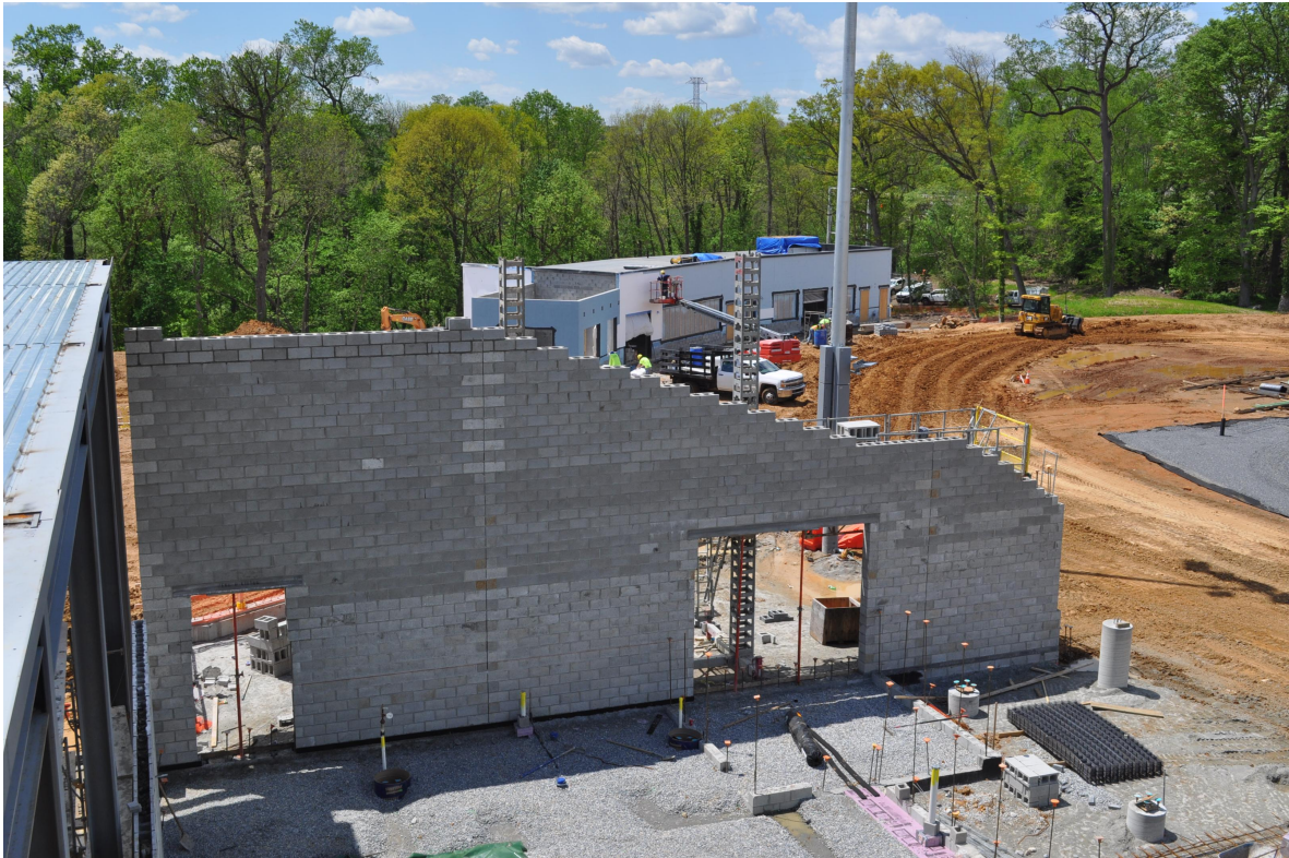
Freestanding Masonry Screen Wall Construction with Concourse Building Construction in Background
