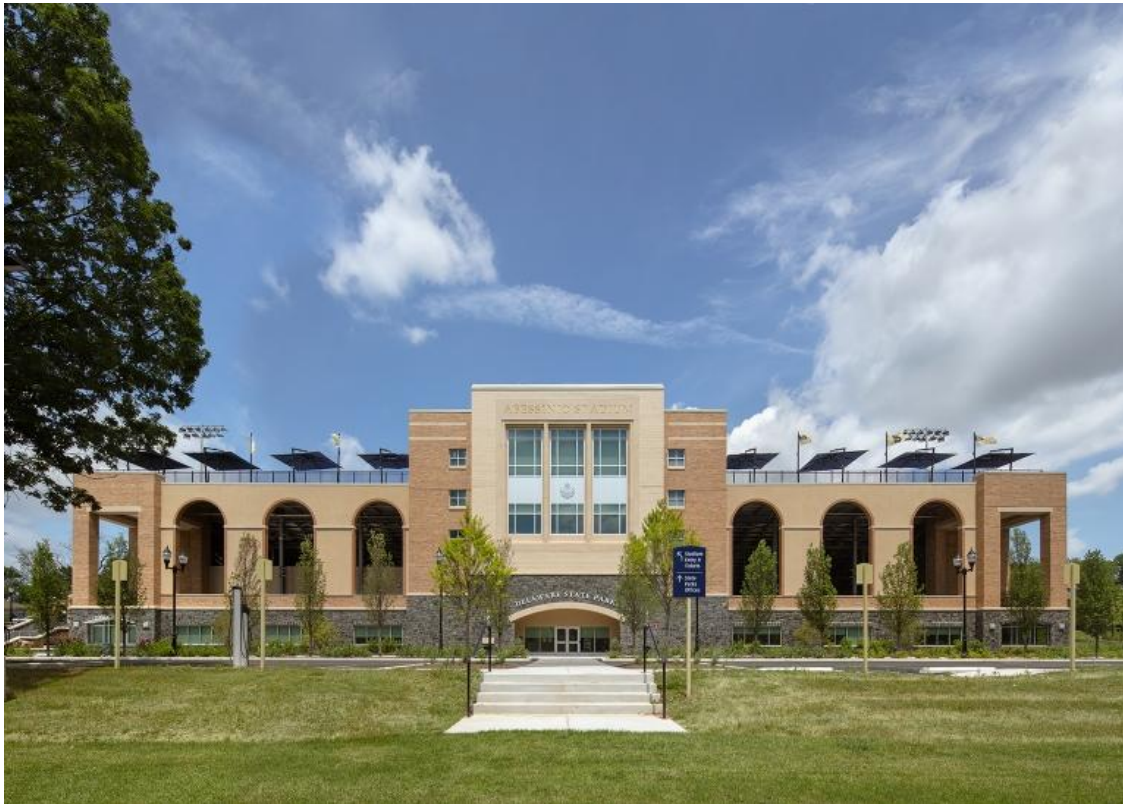
Grandstand Building South Elevation
