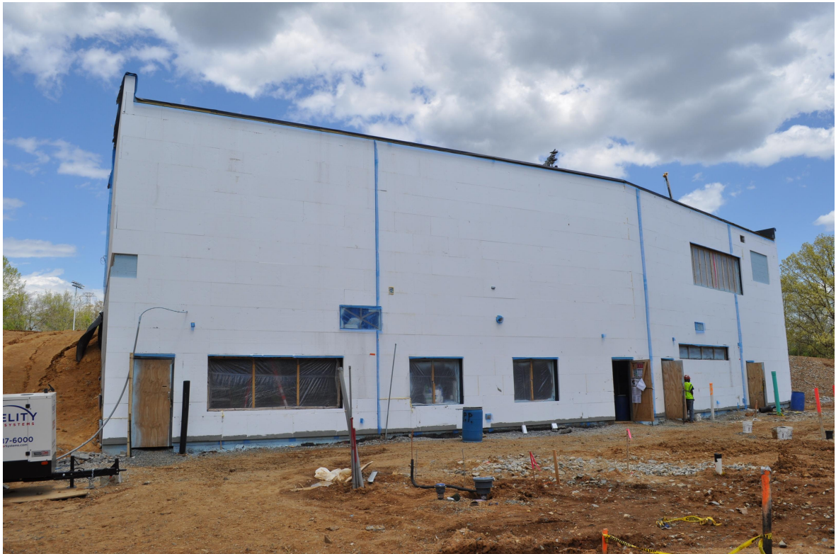
Concourse Building South Elevation Construction
