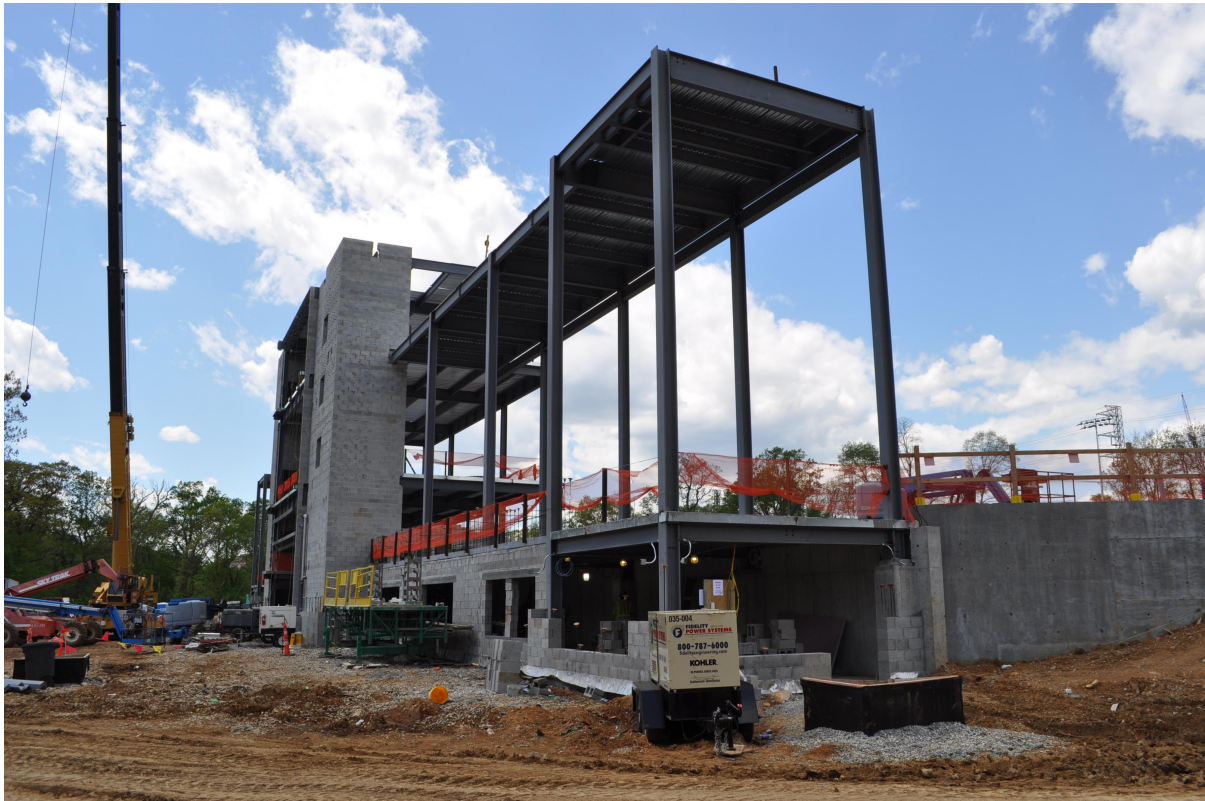
Grandstand Building Southeast Elevation Construction
