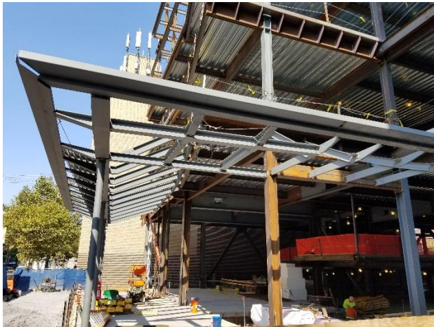
Above Left: Canopy moves from a "v" shaped profile to a more shallow tapered section with over framing Above Right: Over framing as the canopy turns the corner around the building
