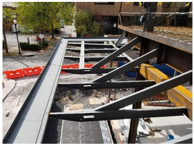
Above Left: Canopy moves from a "v" shaped profile to a more shallow tapered section with over framing Above Right: Over framing as the canopy turns the corner around the building
