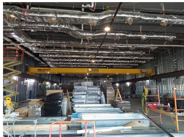
AREA F - FIT OUT LONG SPAN CRANE BAY 1
