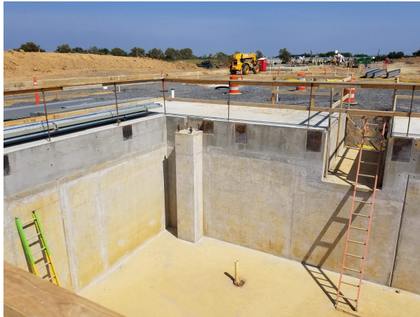
FOUNDATIONS - AREA A DEPRESSED PUMP ROOM
