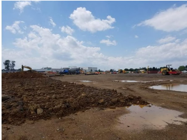
SITE EXCAVATION VIEW FROM SW CORNER OF BLDG
