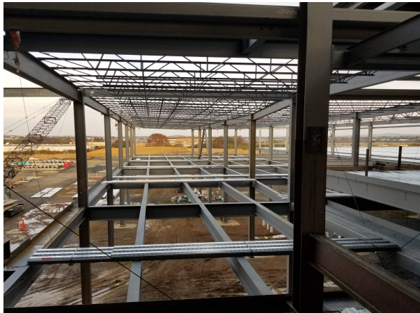
AREA B - STEEL CONSTRUCTION MECHANICAL PLATFORMS AND ROOF
