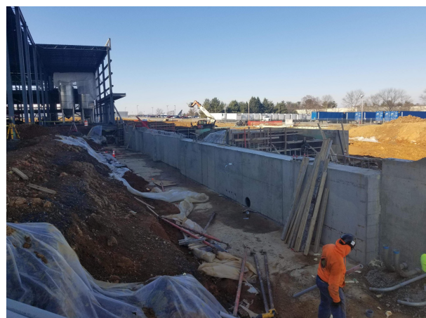
FOUNDATIONS - AREA C COMBINED FOUNDATIONS - MAT SLAB
