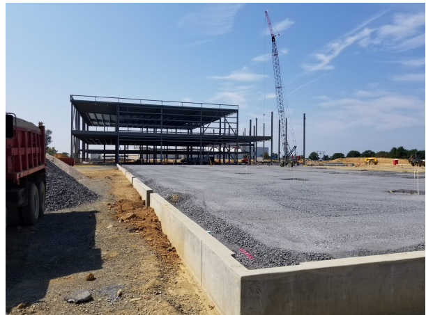
CONSTRUCTION PROGRESS VIEW FROM SW CORNER OF BLDG
