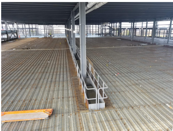
AREA F - SECOND FLOOR ABV CRANES COMPOSITE SLAB CONSTRUCTION
