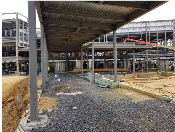
CONNECTING LINK CONSTRUCTION - SE VIEW
