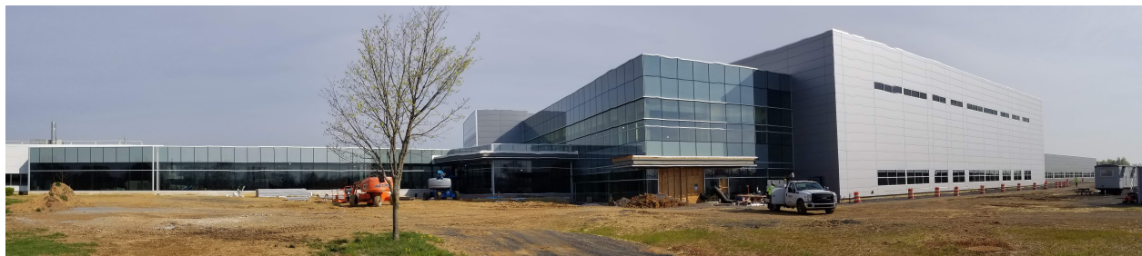
EXTERIOR FACADE CONSTRUCTION VIEW FROM SE CORNER
