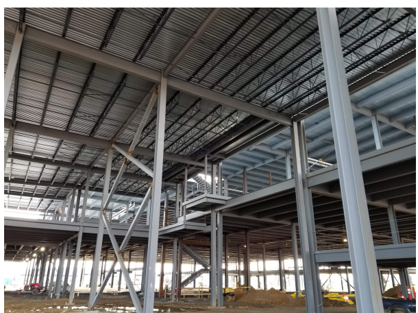
AREA B - VIEW TO PLATFORM AND AREA A MECHANICAL LEVELS
