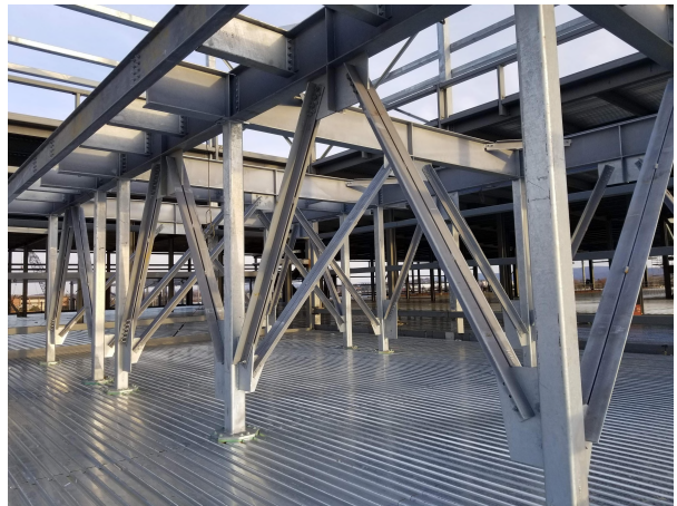
EXTERIOR VIEW - AREA A ELEVATED DUNNAGE PLATFORM
