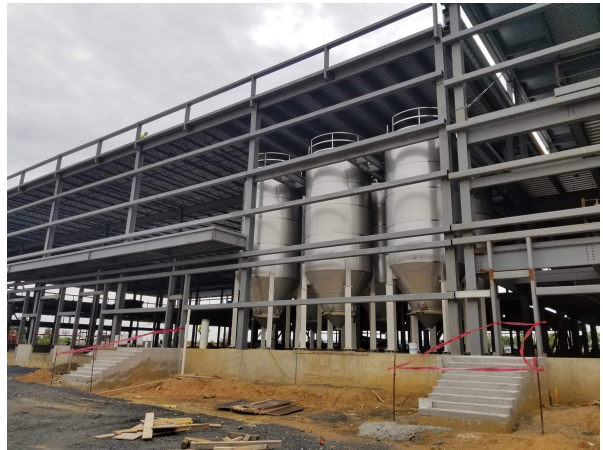
EXTERIOR VIEW - AREA B STEEL CONSTRUCTION AND TANKS
