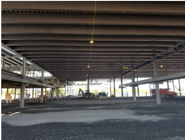
AREA F - STEEL CONSTRUCTION LONG SPAN CRANE BAY 1
