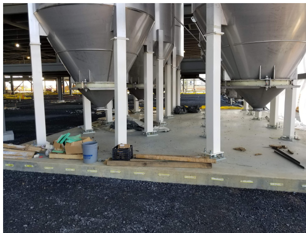
FOUNDATIONS - AREA B PROCESS TANK MAT SLAB
