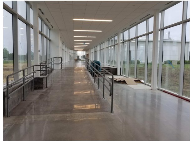
CONNECTING LINK INTERIOR - SW VIEW
