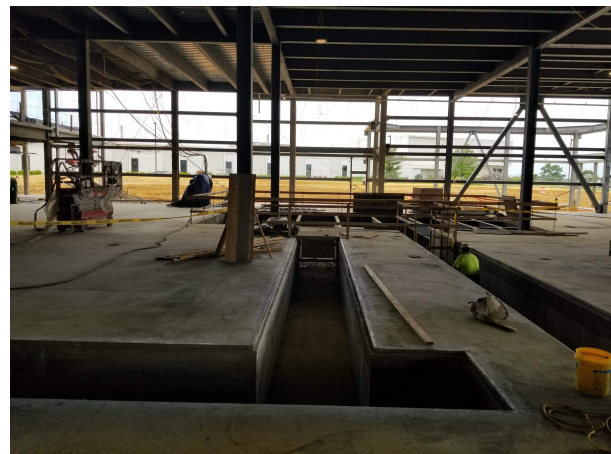
FOUNDATIONS - AREA A SLAB ON GRADE PROCESS TRENCHES
