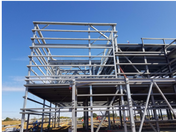
EXTERIOR VIEW - AREA A STEEL CONSTRUCTION
