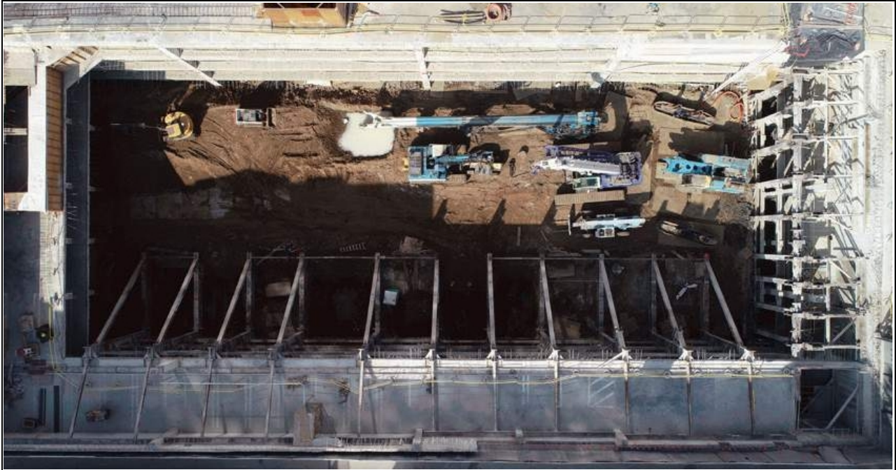
Temporary Support of Excavation Bracing Prior to Start of New Foundations
