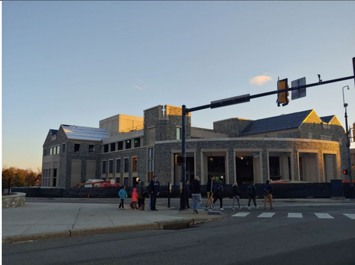
Front Photo (from Ithan Ave) - Skin Complete
