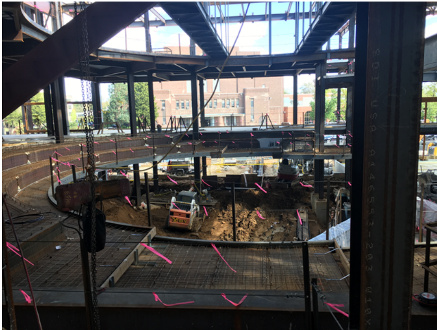
Proscenium Theater Curved, Cantilevered, Stepped Balcony Construction
