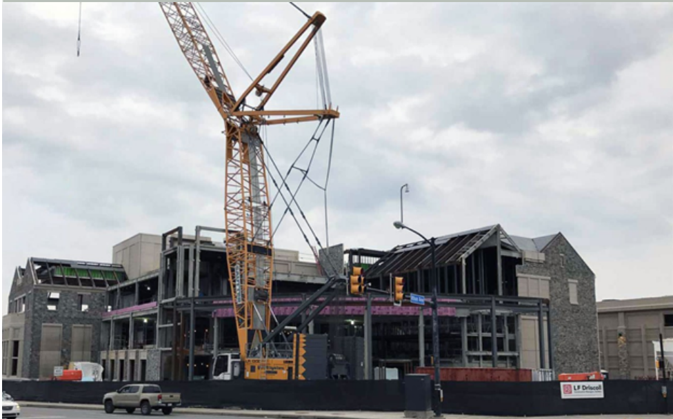
Front Photo (from Ithan Ave) - Steel Complete
