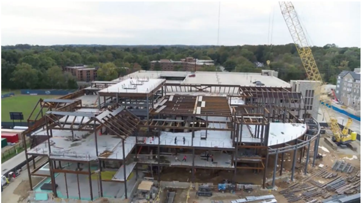
Aerial Photo During Construction
