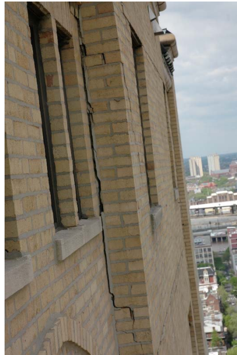
Figure 5 & 6: Cracking at building corners and between panel setbacks.
