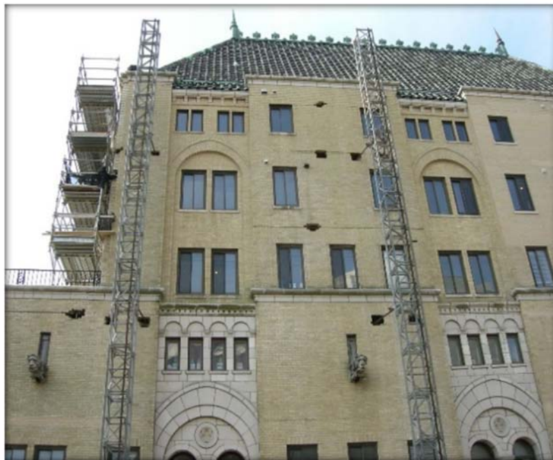
Figure 3: Mast Climber and pipe scaffolding along upper levels of north elevation.
