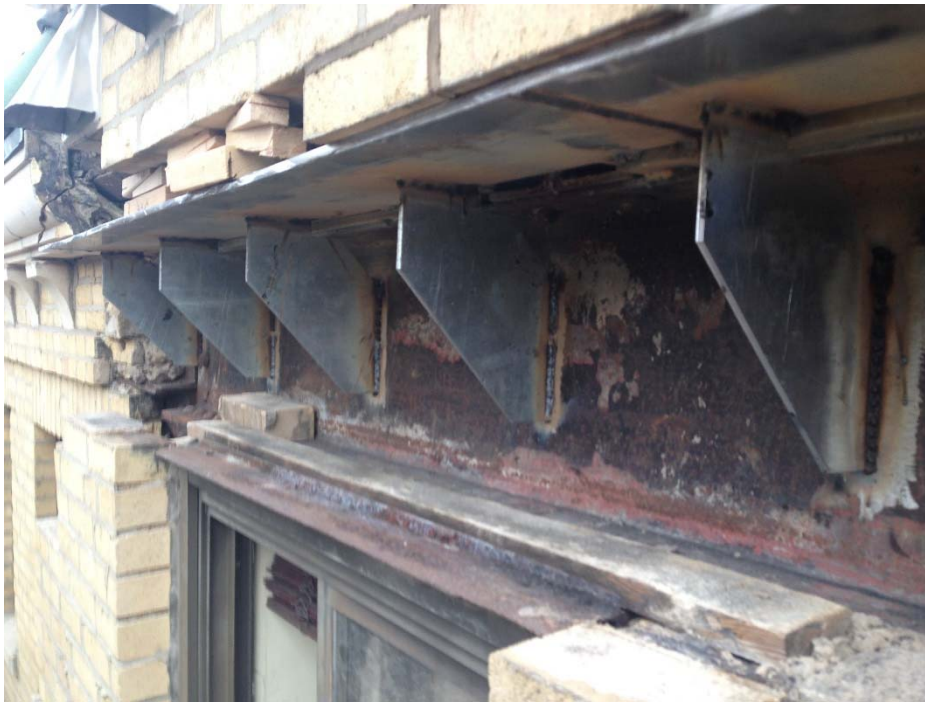
Figure 8: Spandrel beam repair with new steel plate and web brackets.
