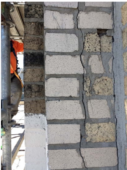
Figure 5 & 6: Cracking at building corners and between panel setbacks.
