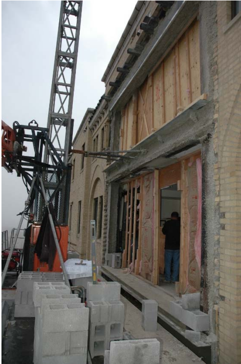
Figure 9: Reconstruction of the top two wall panels below the roof cornice.
