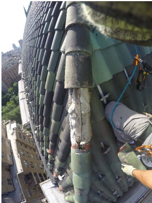
Figure 11: Replacing roof tiles along the hip.
