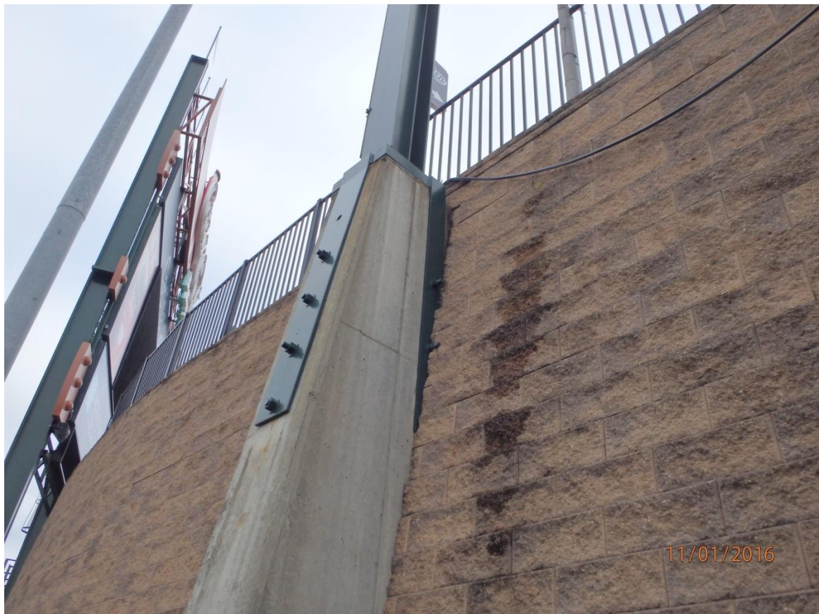
Ad board typical column base plate strap attachment to concrete pier.
