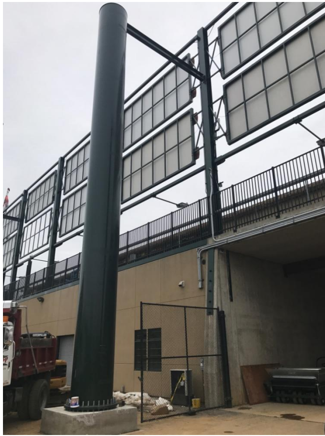
Typical pipe shoring post installed to brace existing ad board column.
