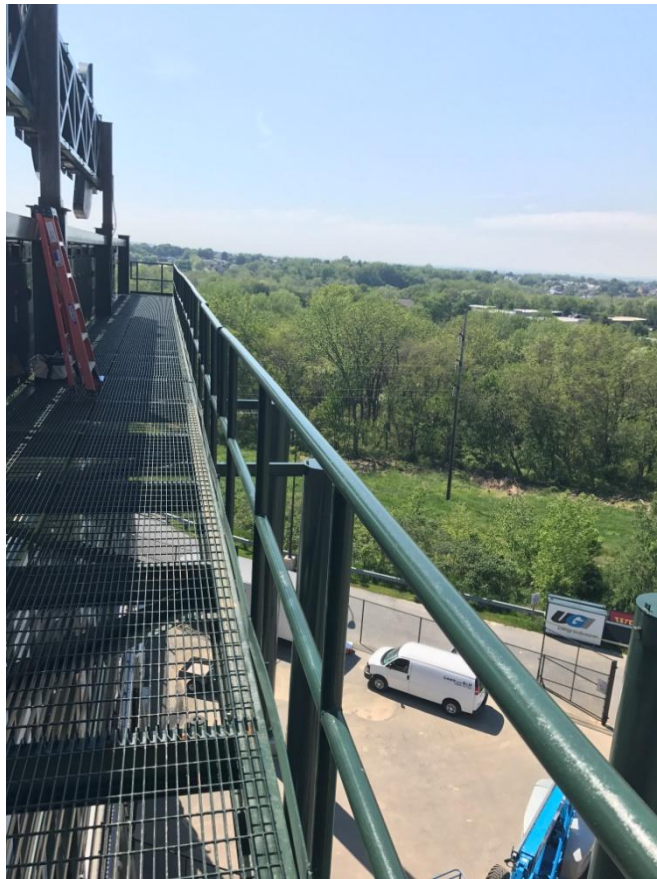
New Service platform.
