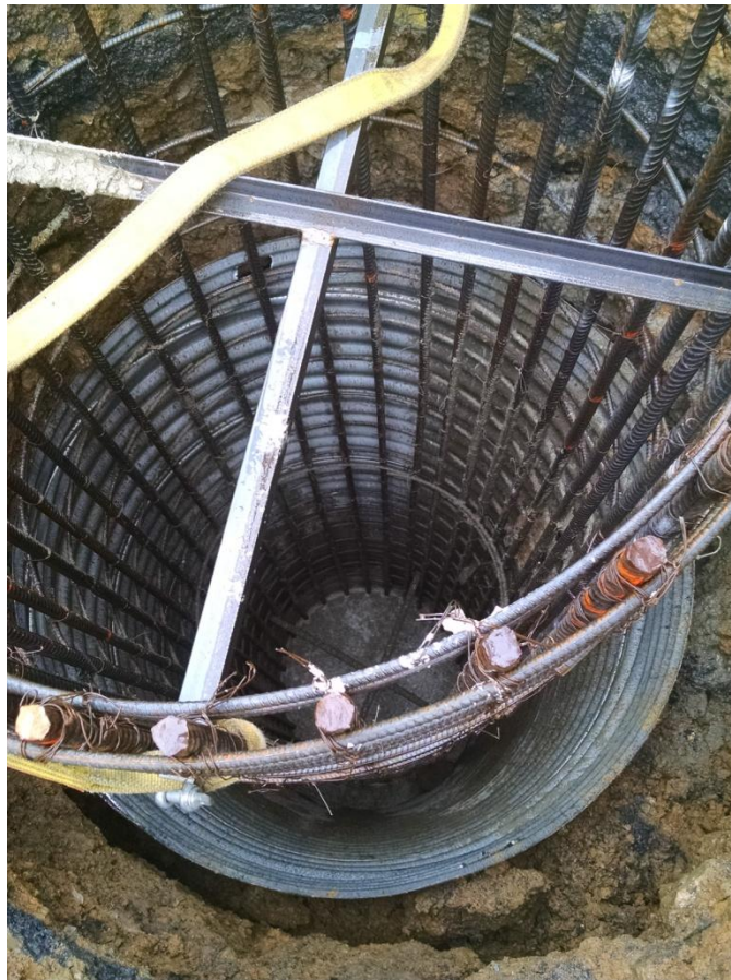
Drilled caisson reinforcing for new pipe shore.
