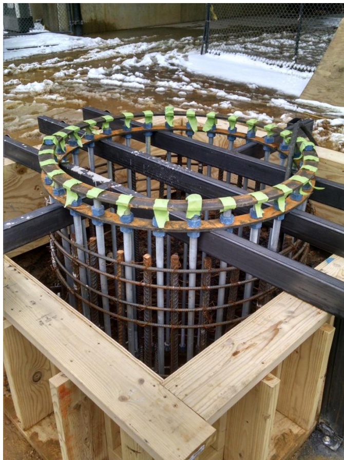
Bolts and caisson reinforcing for new pipe shore.
