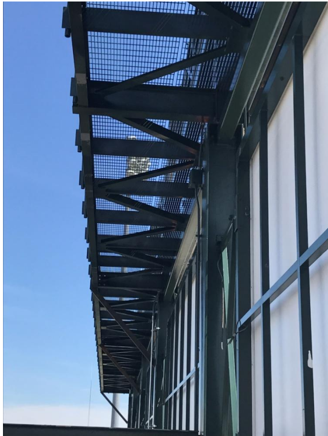
New service platform Steel cantilevered from existing ad board columns.
