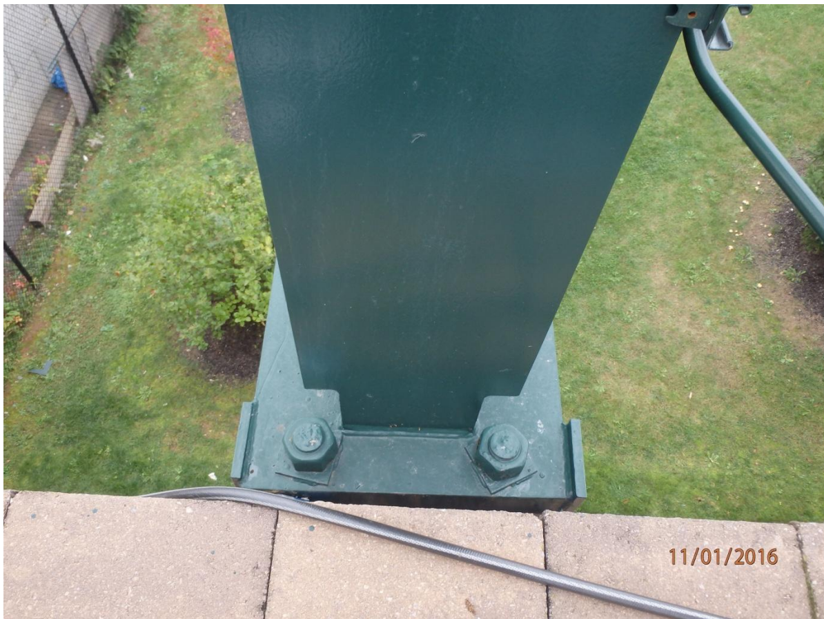
Ad board typical column flange cope at base plate attachment to concrete pier.
