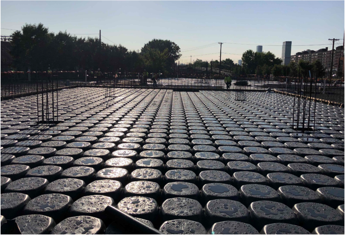
CUPOLEX FORMS FOR DETENTION BASIN
