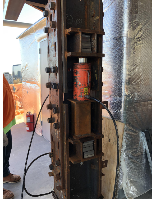
Penn Pavilion North End Level 9-10 Column Splice Detail - Jacking Setup Before & During (Splice Bolts Loose)
