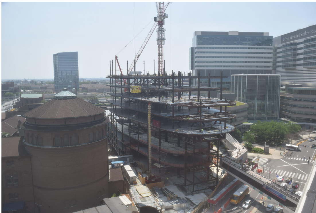
Penn Pavilion Cantilevered North End Truss Temporary Shoring Tower - Aerial View
