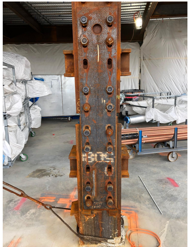
Penn Pavilion North End Level 9-10 Column Splice Detail - Shimmed Gap & Tightened Bolts During Erection
