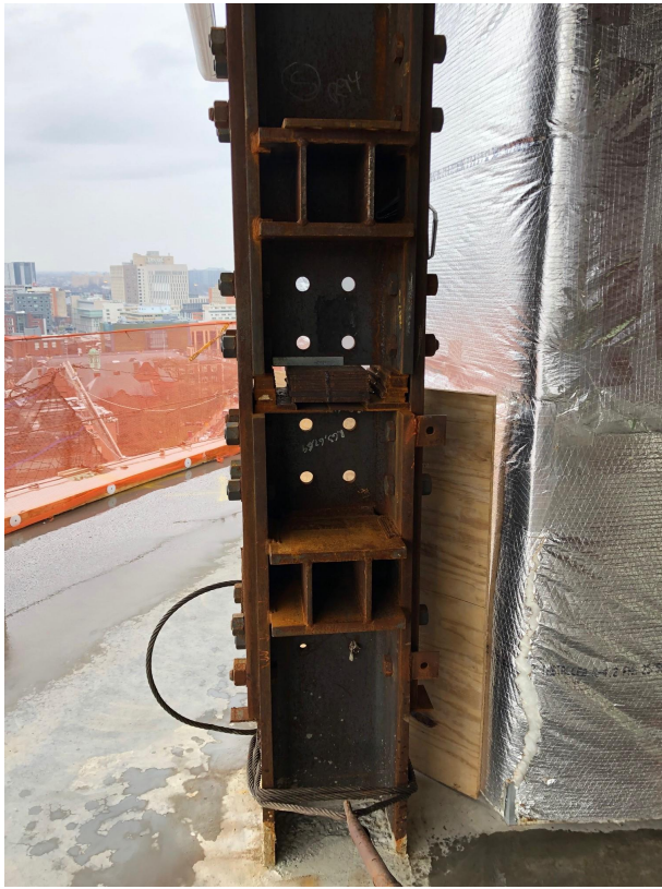
Penn Pavilion North End Level 9-10 Column Splice Detail - Shimmed Gap & Tightened Bolts During Erection
