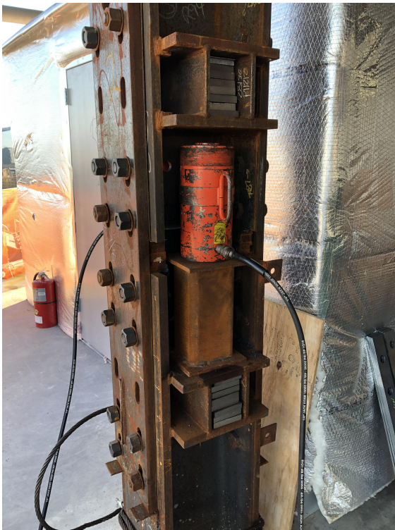
Penn Pavilion North End Level 9-10 Column Splice Detail - Jacking Setup Before & During (Splice Bolts Loose)
