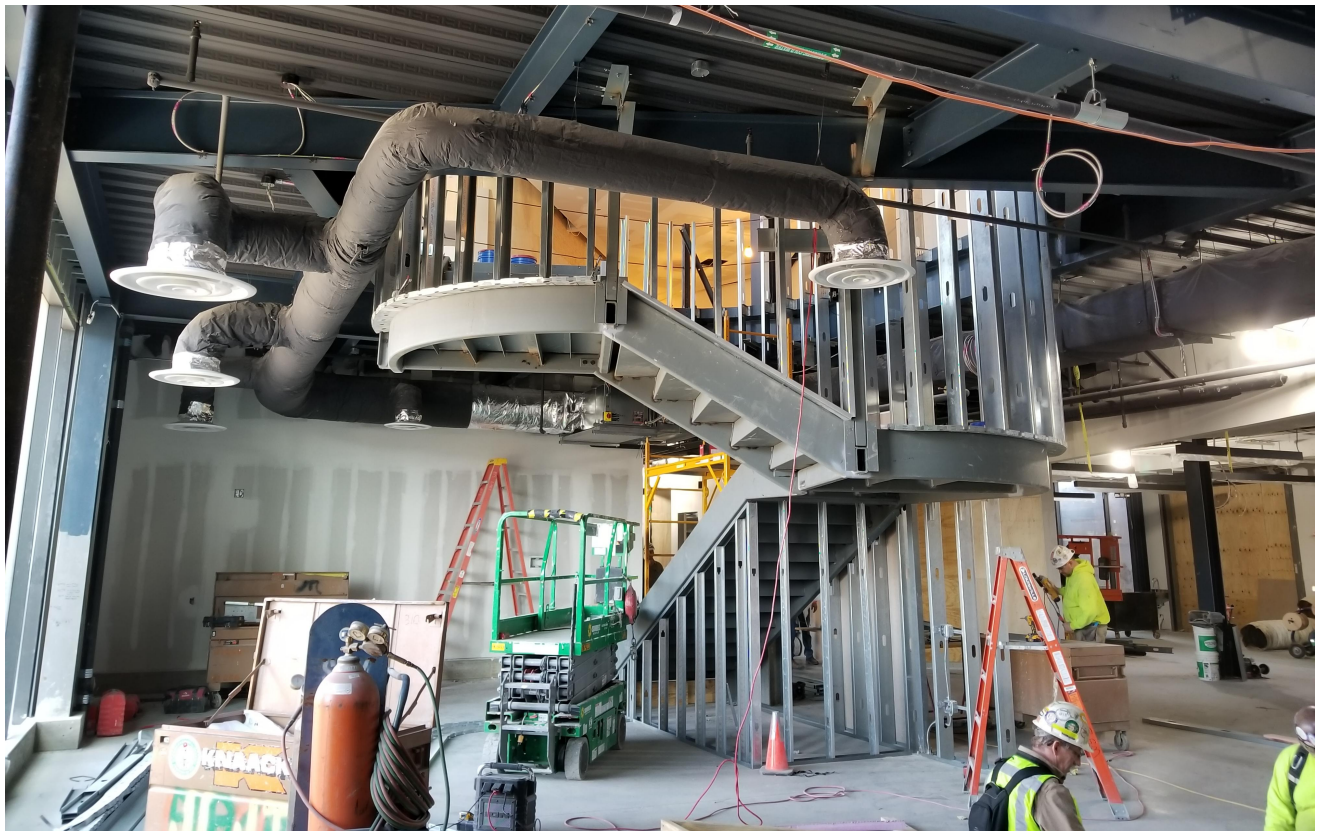
Below - One of the three internal communicating staircases. This stair is suspended from the second floor framing and is composed of curved HSS members and stringers.
