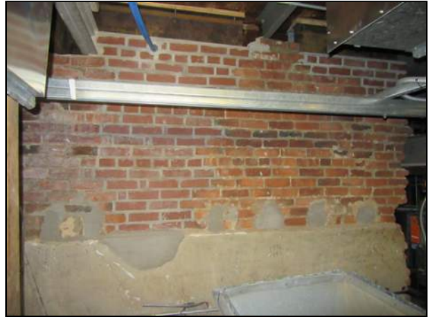
Before and after - bearing wall improvements in attic to support scaffolding loads.
