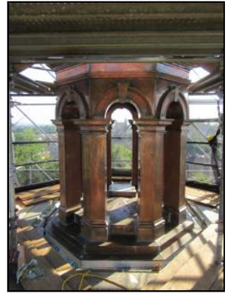
New copper cladding installed to match original.
