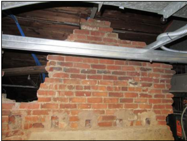
Before and after - bearing wall improvements in attic to support scaffolding loads.
