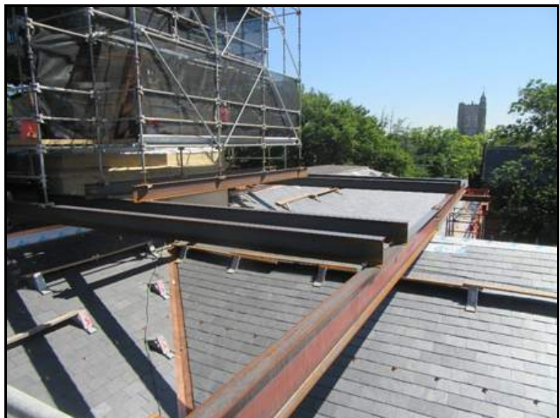
Before and after - bearing wall improvements in attic to support scaffolding loads.
