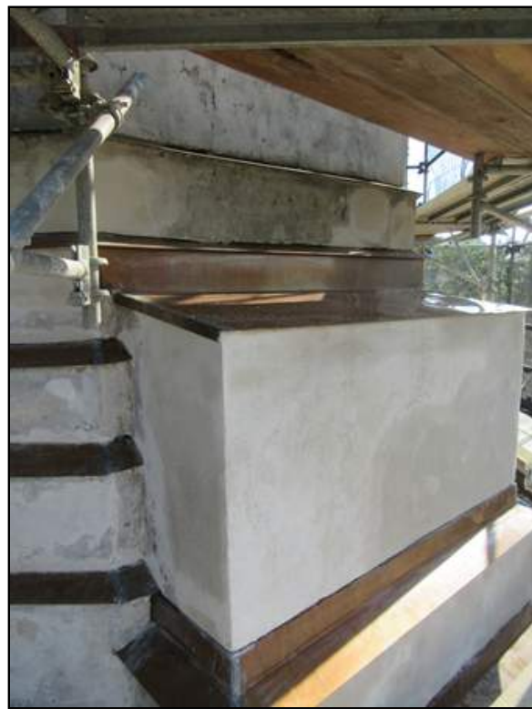
Brick masonry and stucco repairs in progress.
