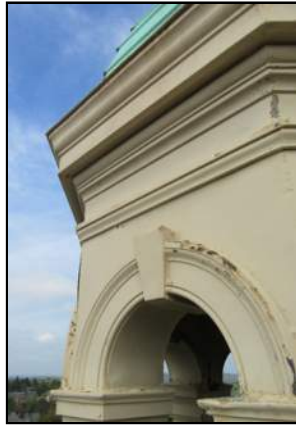
New copper cladding installed to match original.
