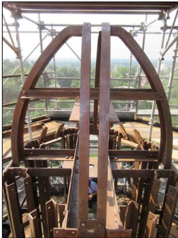
Iron frame rehabilitation in progress.
