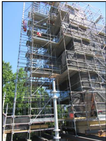
Bell tower scaffolding bridging main roof.
