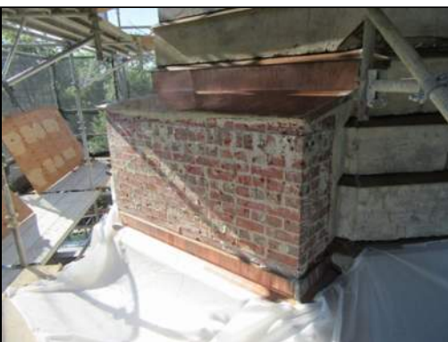
Brick masonry and stucco repairs in progress.
