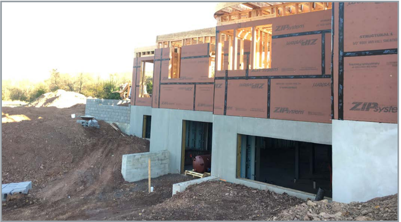
PRECAST CONCRETE WALL PANELS AT WALKOUT BASEMENT AREA
