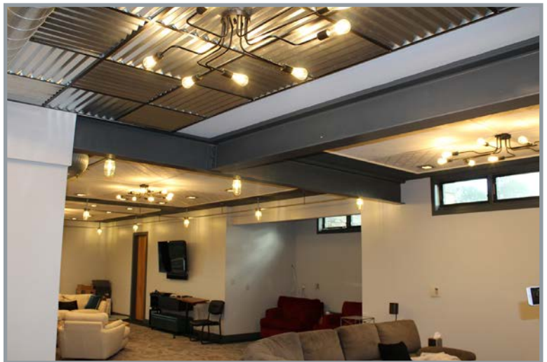
PHOTO OF STEEL BEAMS INTEGRATED WITH ROOM DÉCOR
