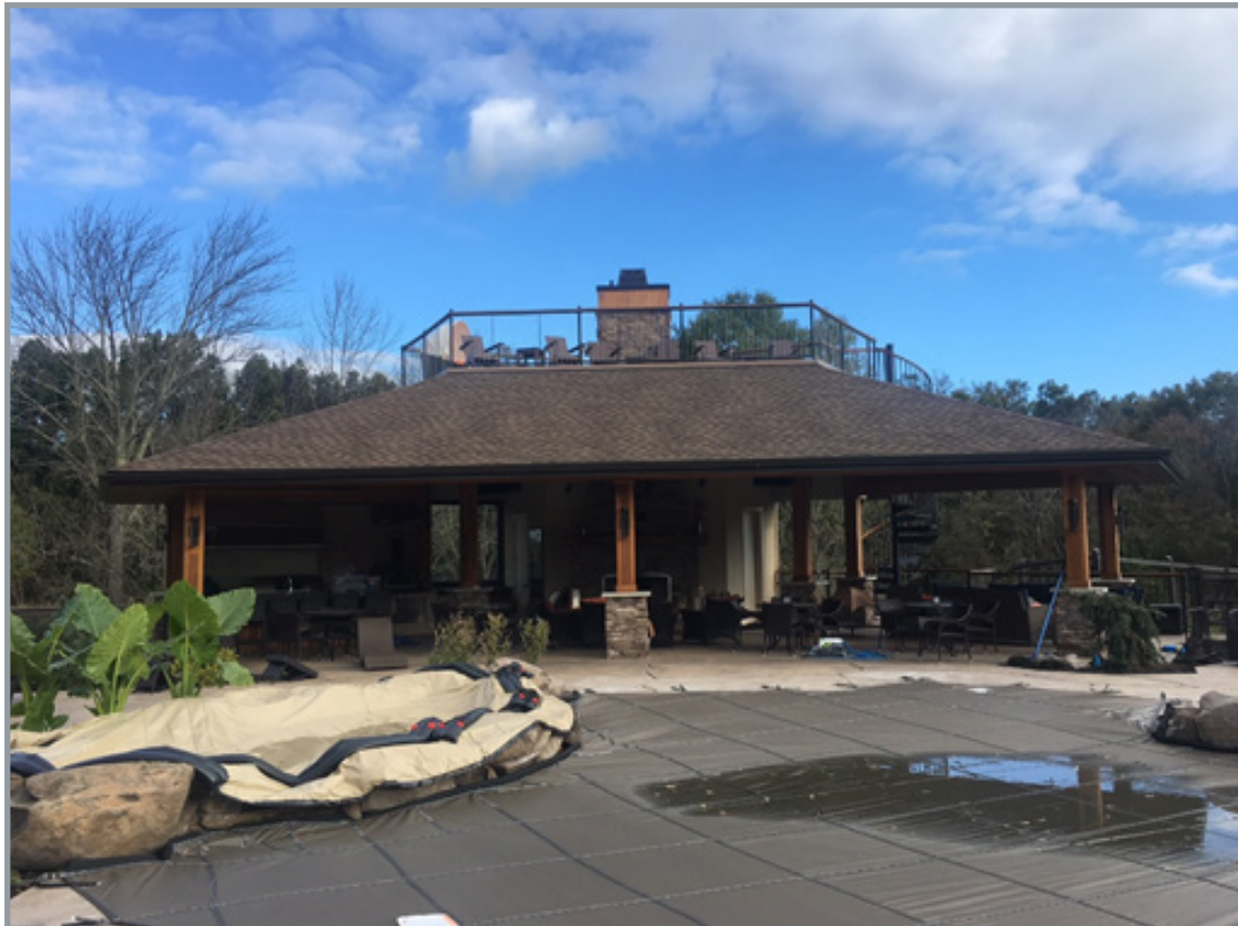
PHOTO OF FINAL LOOK OF POOL HOUSE
