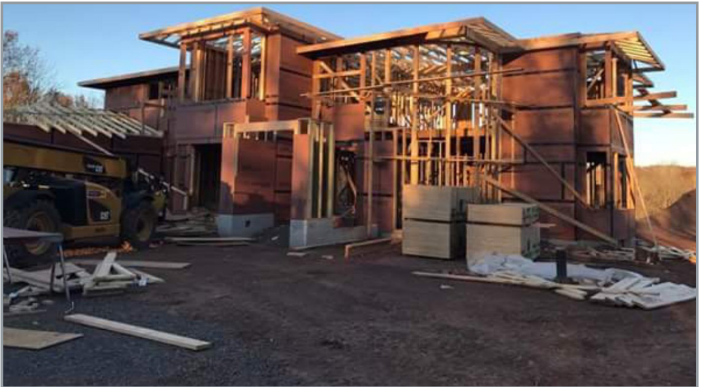
FRONT ENTRANCE - CONSTRUCTION PHASE
