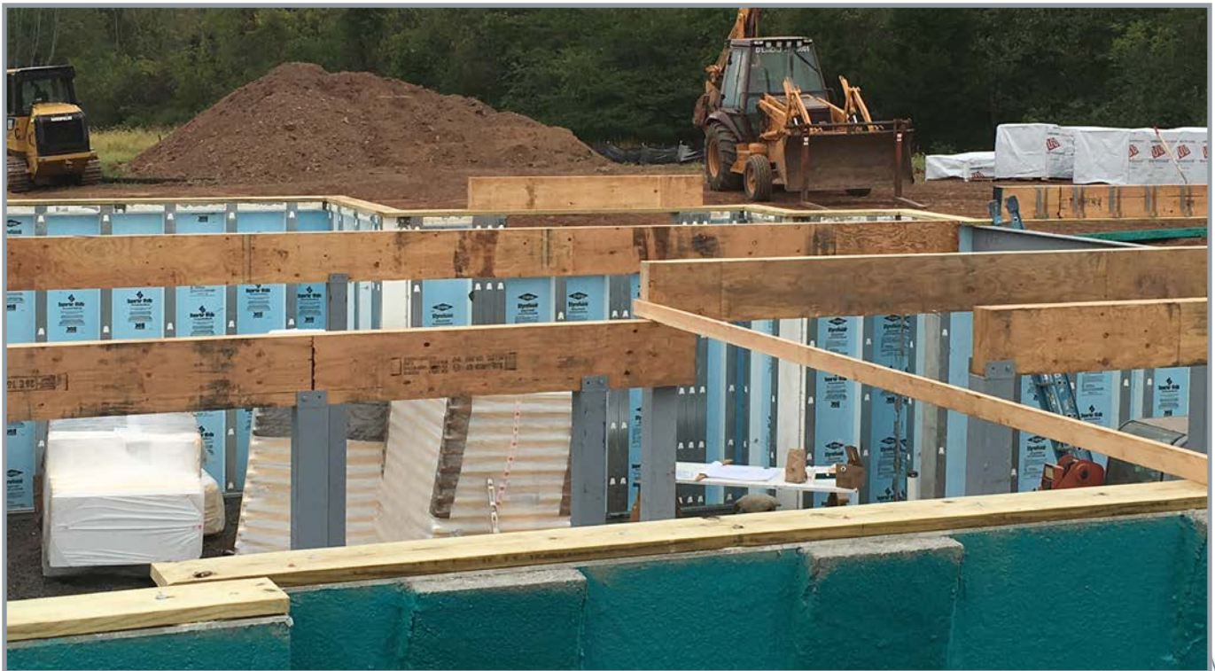
ERECTION OF PRECAST CONCRETE WALL PANELS
