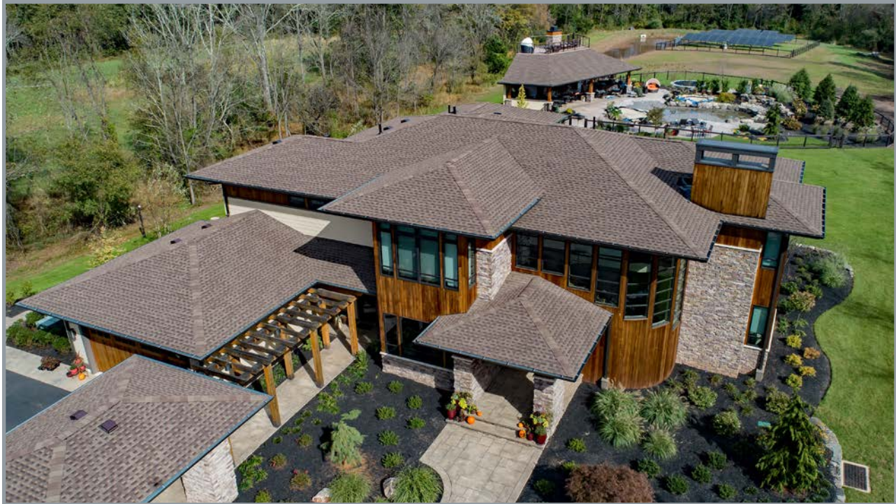
FRONT ENTRANCE - COMPLETED PHASE
