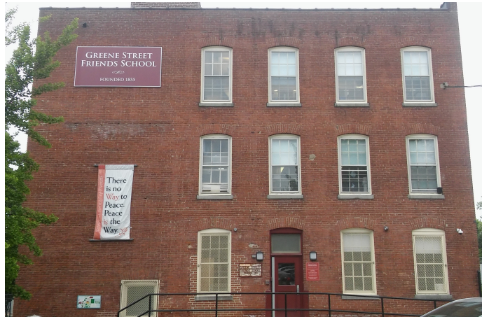
FORMER FACADE AT ARAMAT BUILDING
