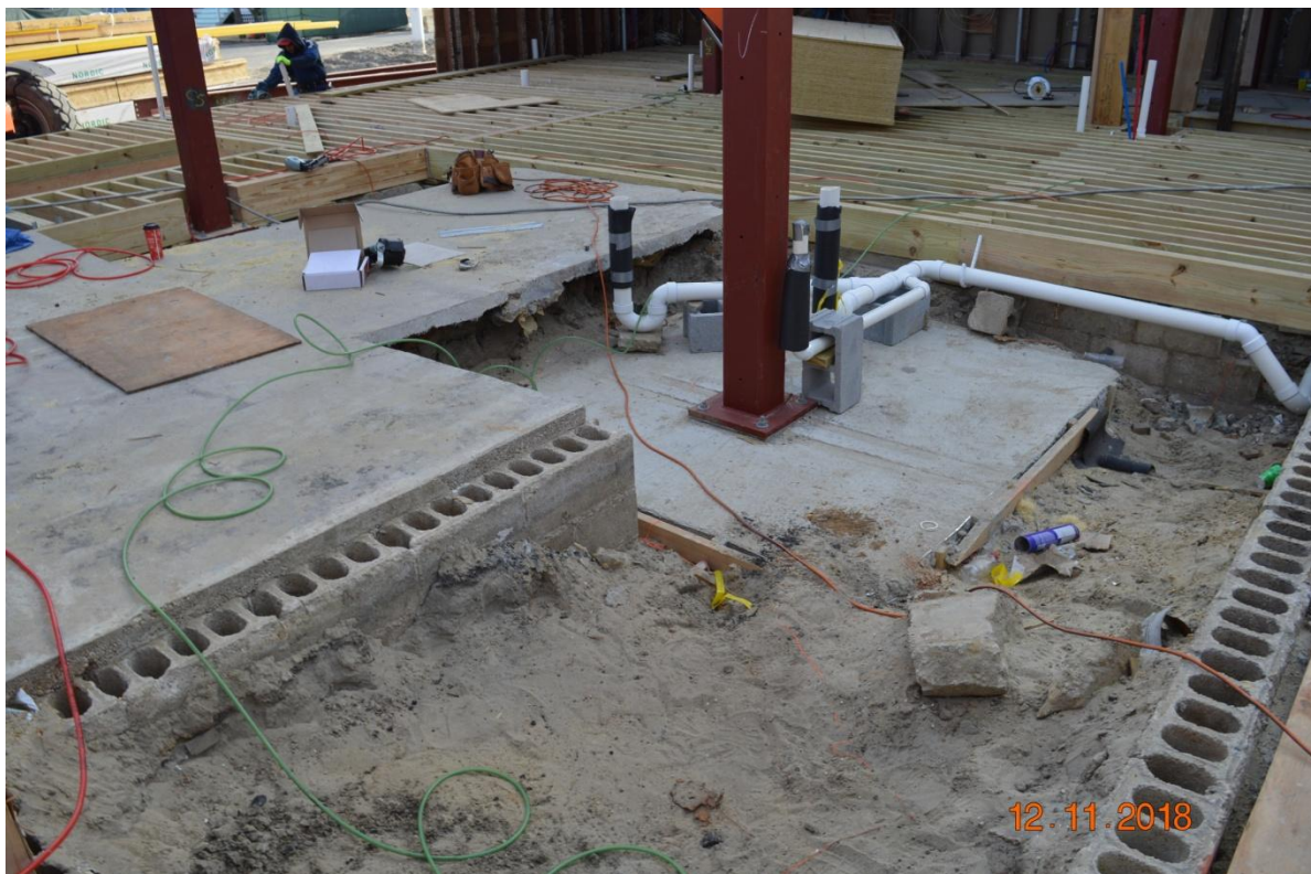
Steel column supported on pile cap in crawl space. New wood framing installed over crawl space to replace rotted floor areas.
