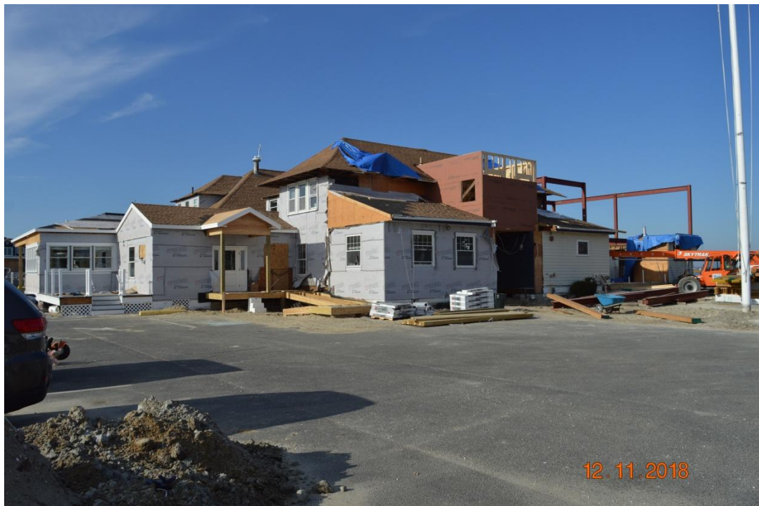
Additions and renovations under construction.
