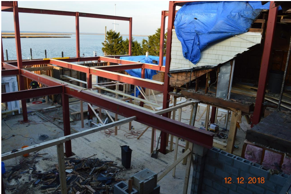
Steel framing for new second floor and roof at addition.
