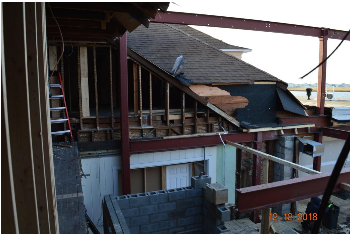
New steel framing being installed around existing wood construction to remain.
