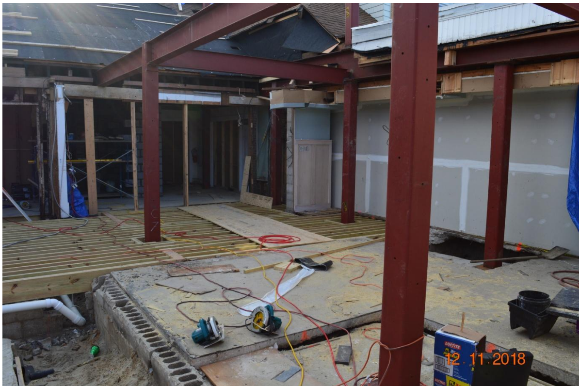
Steel columns for dining room addition installed into crawl space on pile caps.
