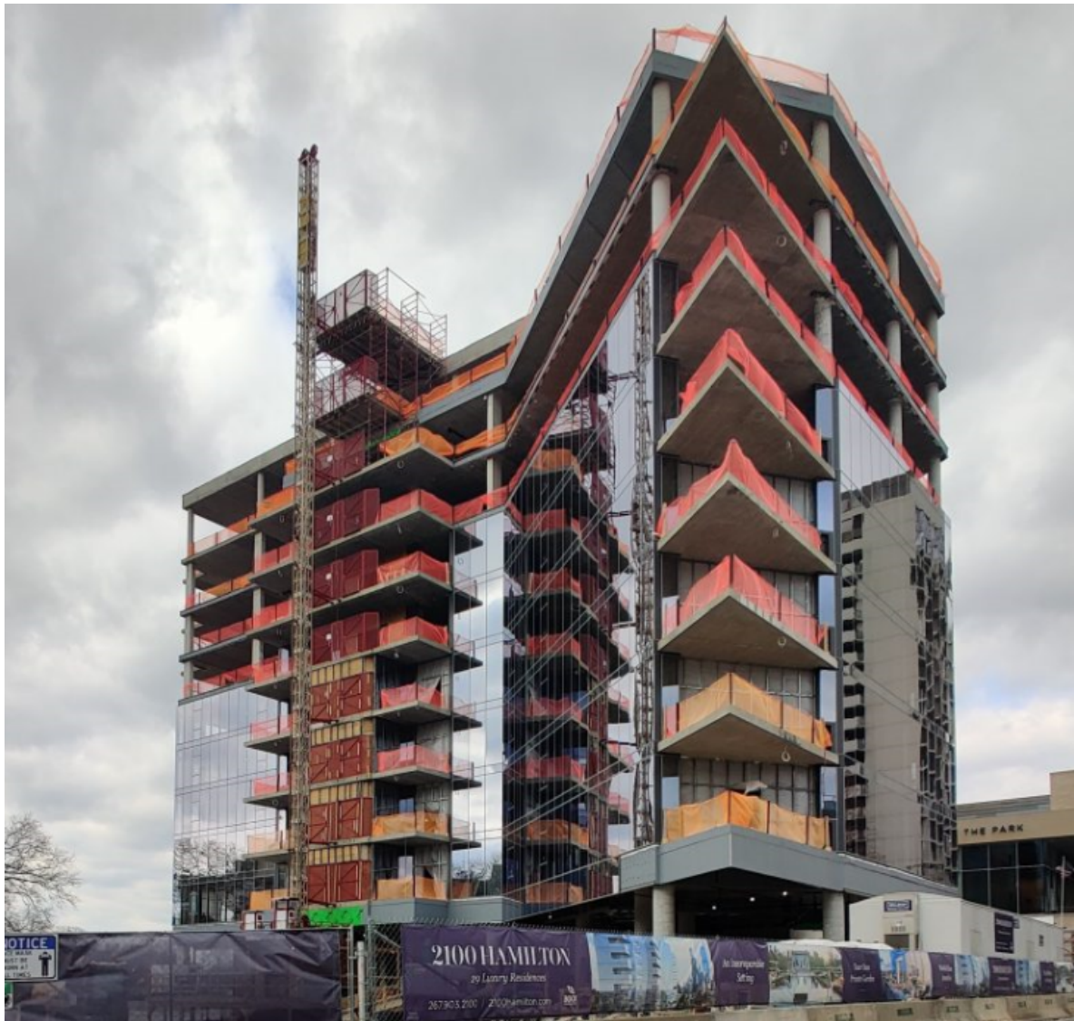
WINDOW WALL INSTALLTION
