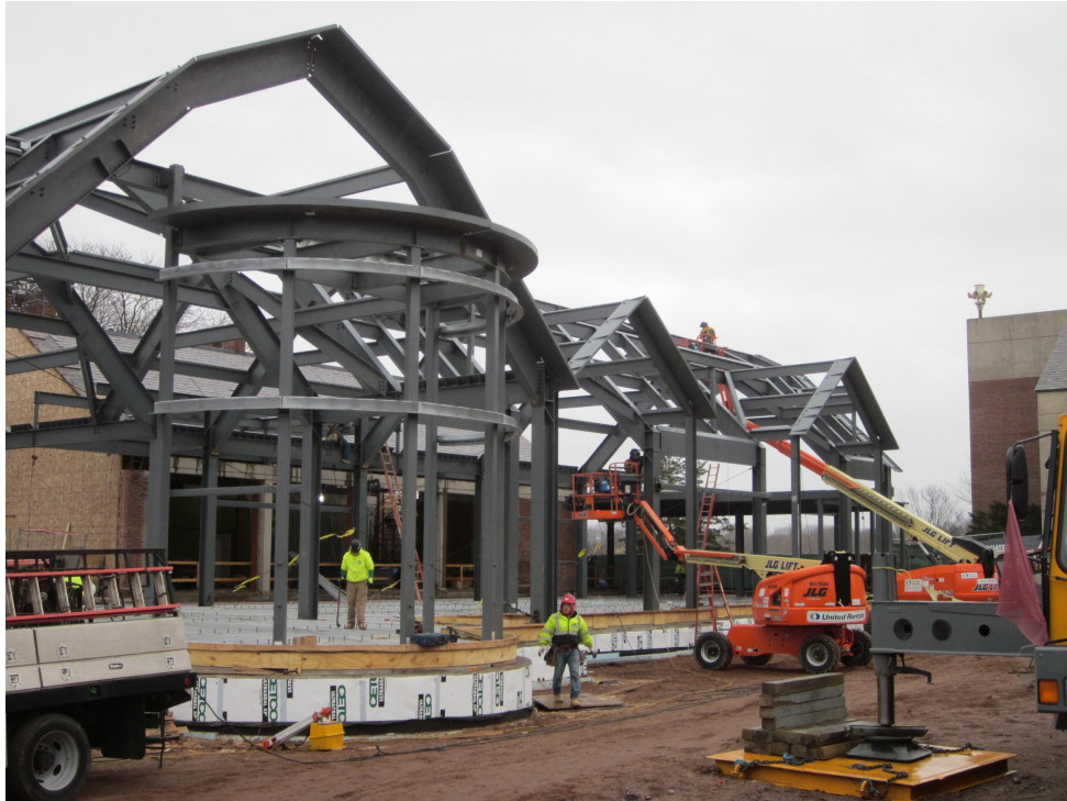
Half round bay framing with supplemental HSS members for support of case stone panels
