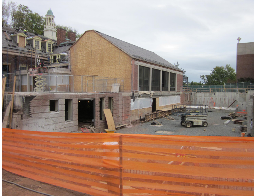
View of South Elevation showing the New Addition Foundation, 1969 Addition (Center), and 1988 Addition demolished to First Floor
