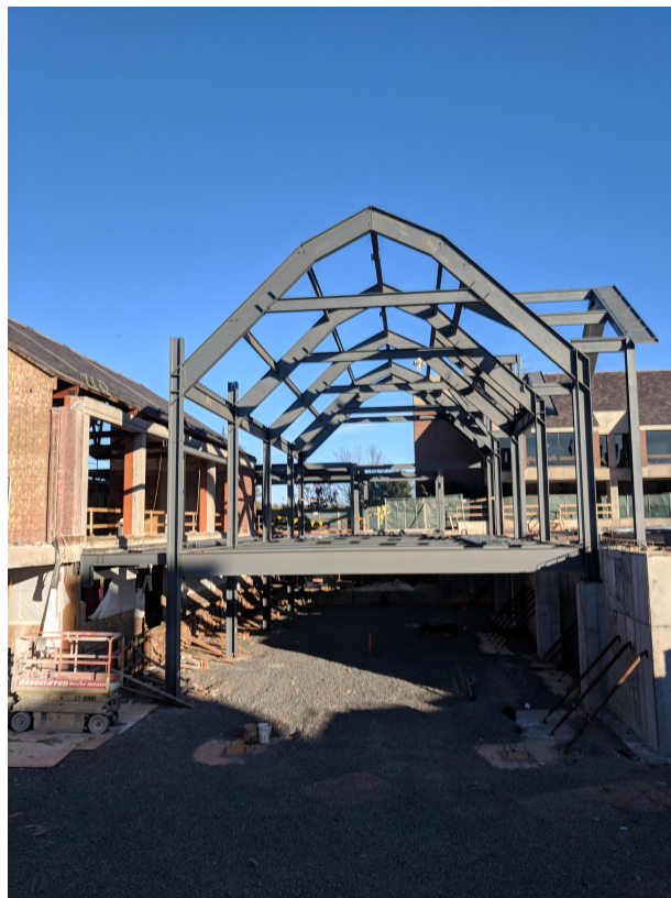
View of New Addition steel framing looking East (existing 1969 Addition on left)
