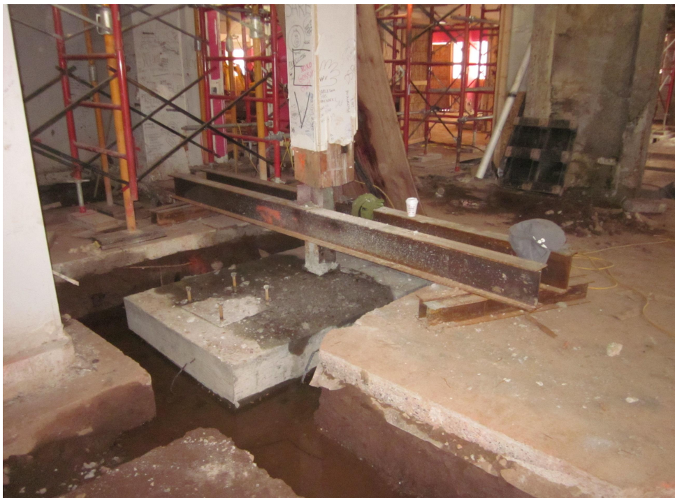
Existing column temporarily shored for installation of new combined footing
