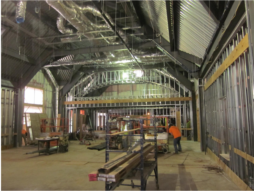
New Addition interior with bent WF24 beams and hangers for barrel vault ceiling
