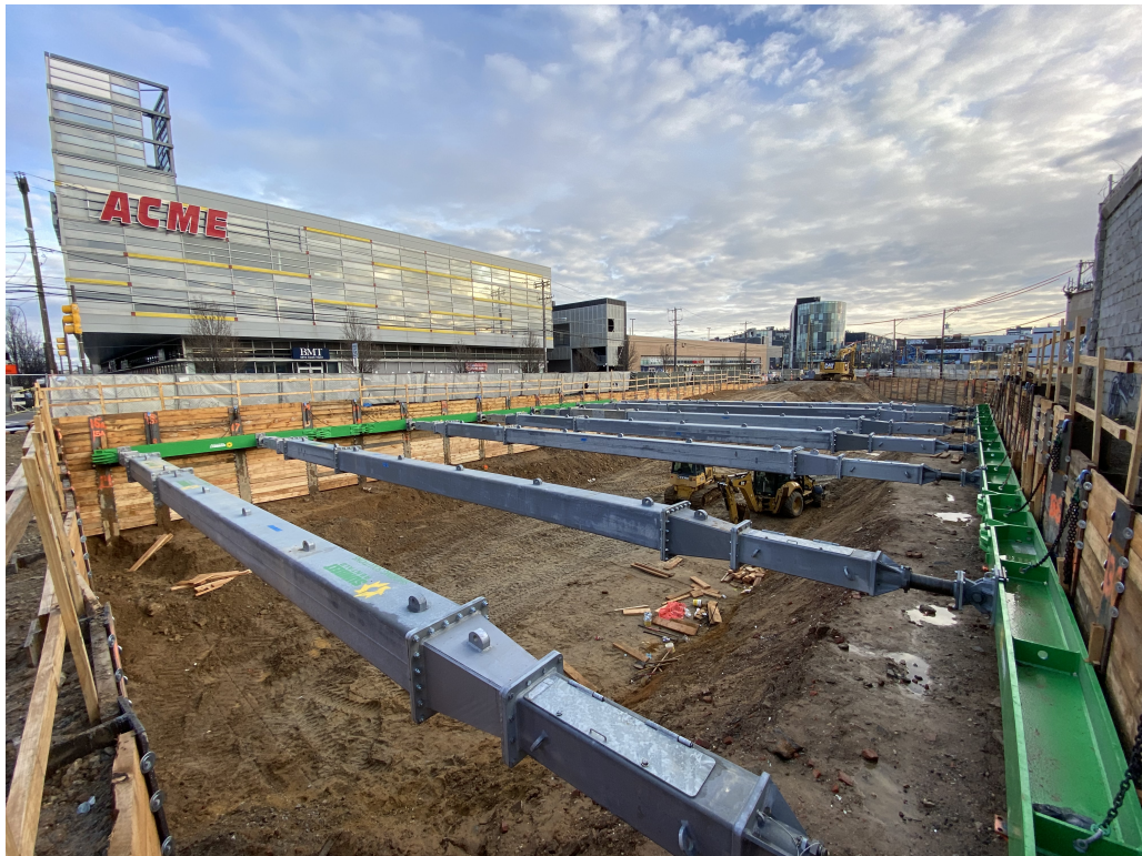
STAGE 1: HEEL BLOCK, UPPER WALERS, & UPPER RAKERS INSTALLATION
