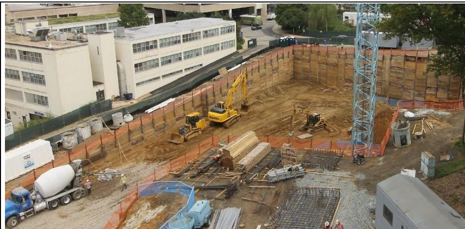
October 2018: Due to the steeply sloped project site, the bottom 2 levels of the building on the southeastern side were constructed below grade with temporary sheeting and soldier piles around the perimeter of the building. The uneven lateral earth pressure on the building structure results in a significant lateral load onto the shear walls in addition to the wind and seismic forces.
