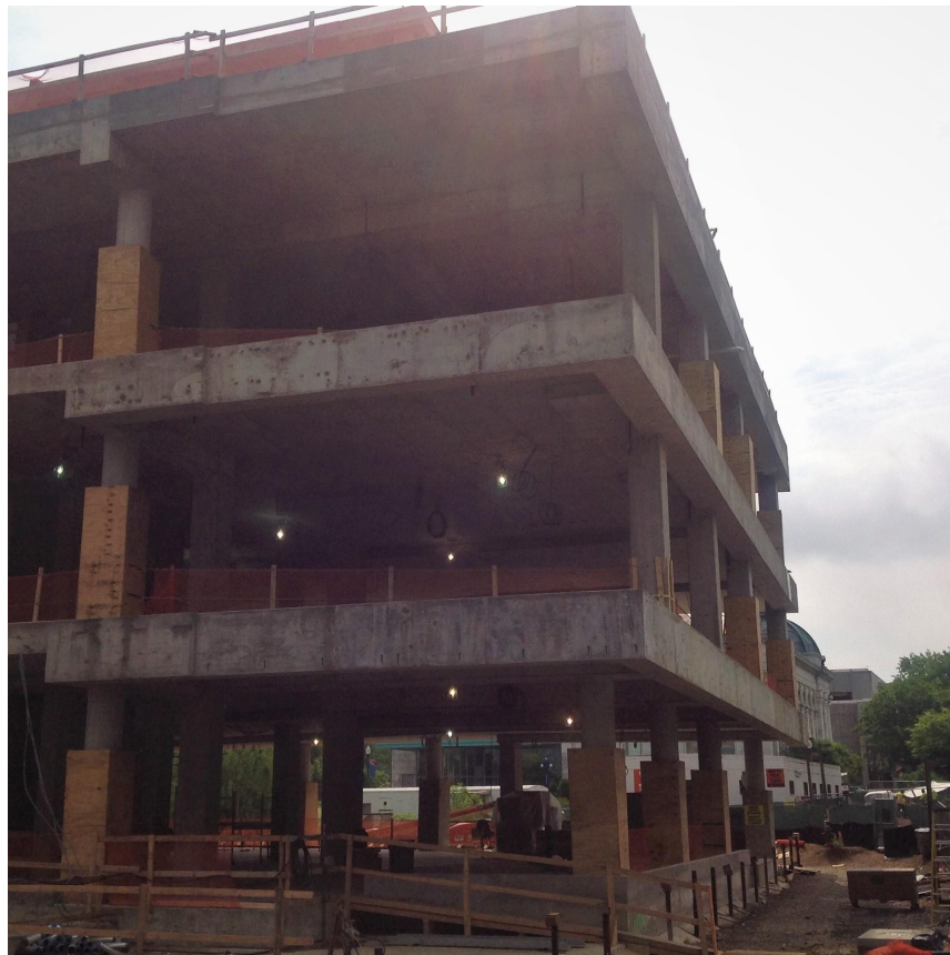
Looking east at the south end of the building, prior to the construction of the masonry facade, where the columns along the south face of the building above the 1st floor level are offset 4'-0" with cantilevered transfer girders. Additionally, the floor slabs in the foreground are cantilevered 15'-0" beyond the column centerline.
