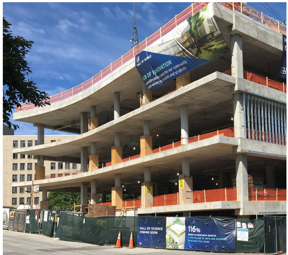
Looking south at the curved east face of the building where the columns are set back 6'-0" from the edge of the slab.
