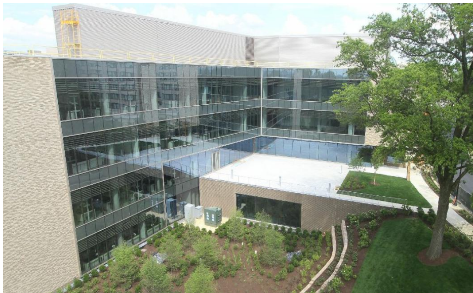
June 2020: The exterior masonry and glass curtain wall facade erection is complete and the roof terrace above the lecture hall is finished.
