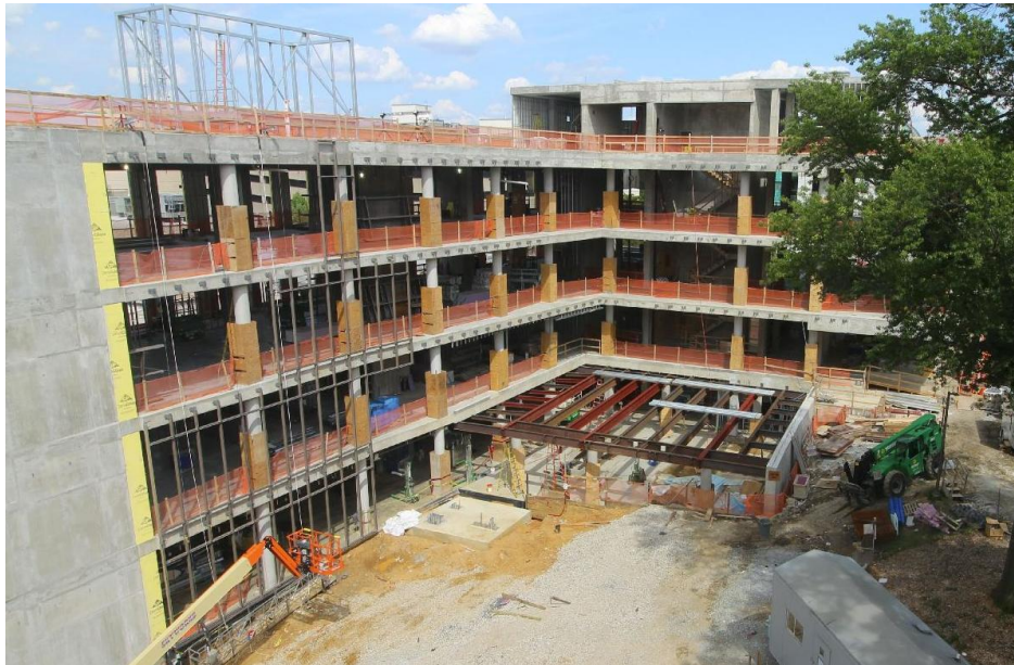
May 2019: The building superstructure was topped out and the concrete gained the required strength to allow for the removal of the shoring. Plywood enclosures are visible around the concrete columns to protect the surfaces that are to be left exposed in the final fitout. The longspan steel framing above the lecture hall to support the roof terrace above is in place.
