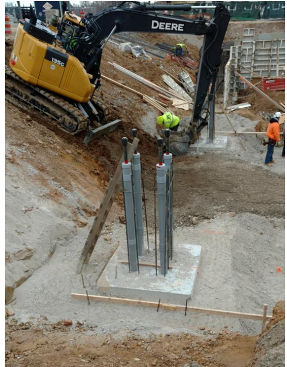
Anchor rods detail and pictured during construction
