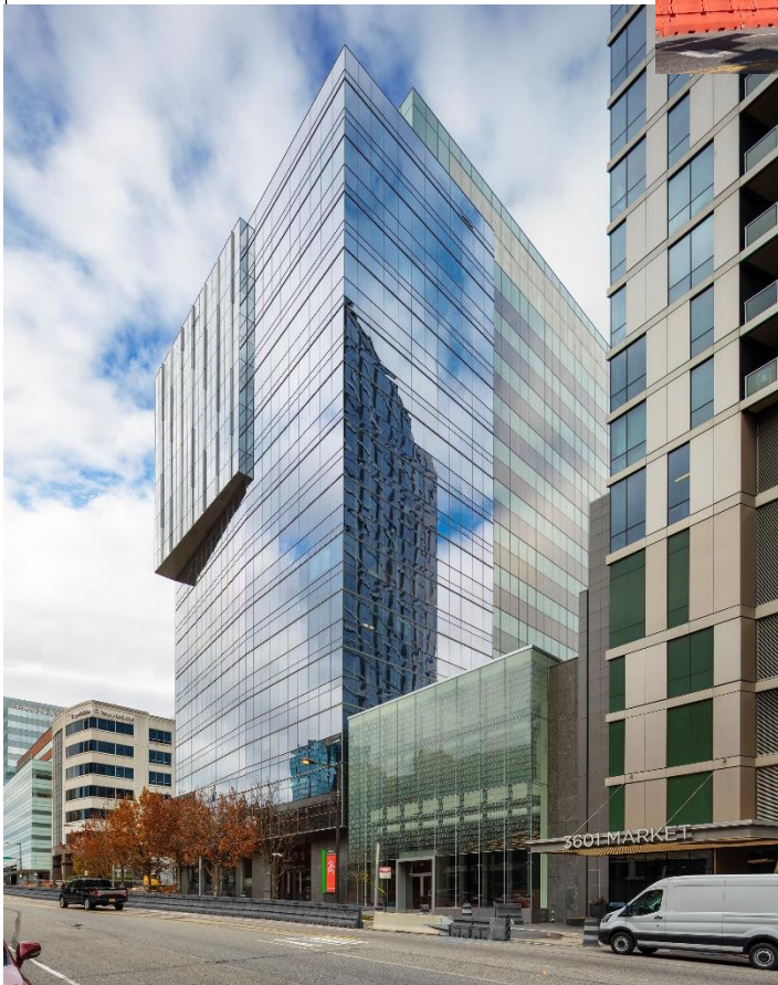
Above: Construction of 3675 Right: 3675 completed with the two story Quorum Space in the foreground.
