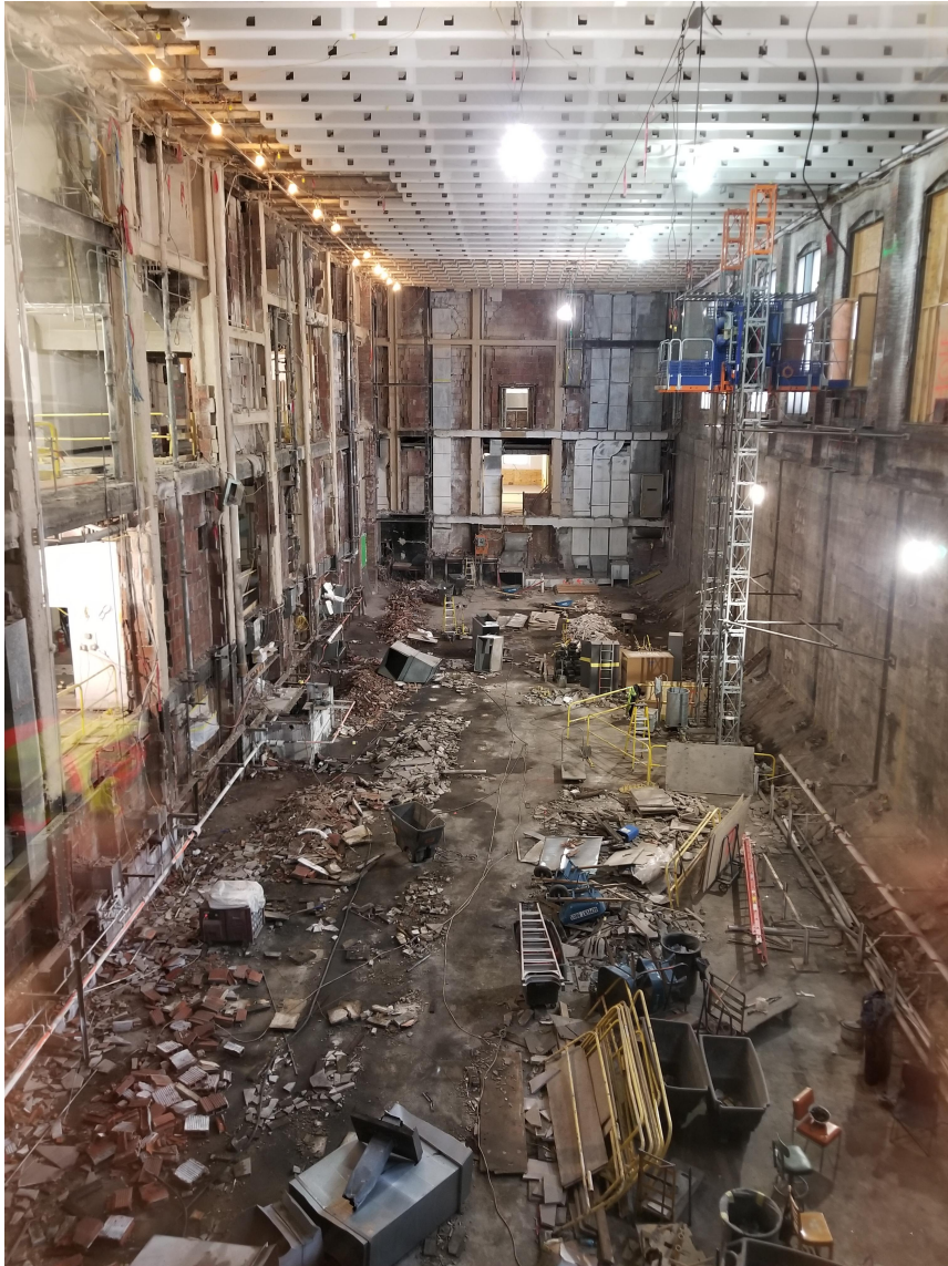
Library Renovation Space Following Stacks Demolition
