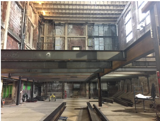
Lower Level Steel Framing Erection
